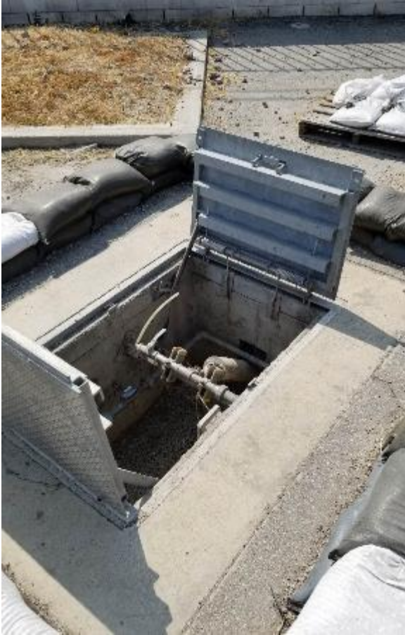
Figure 31. Angled extraction well EW-A. Facing southeast.
