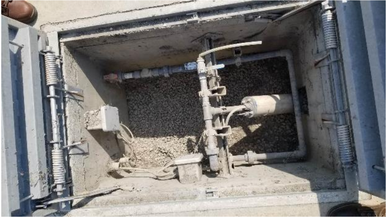
Figure 32. Vault interior EW-A.
