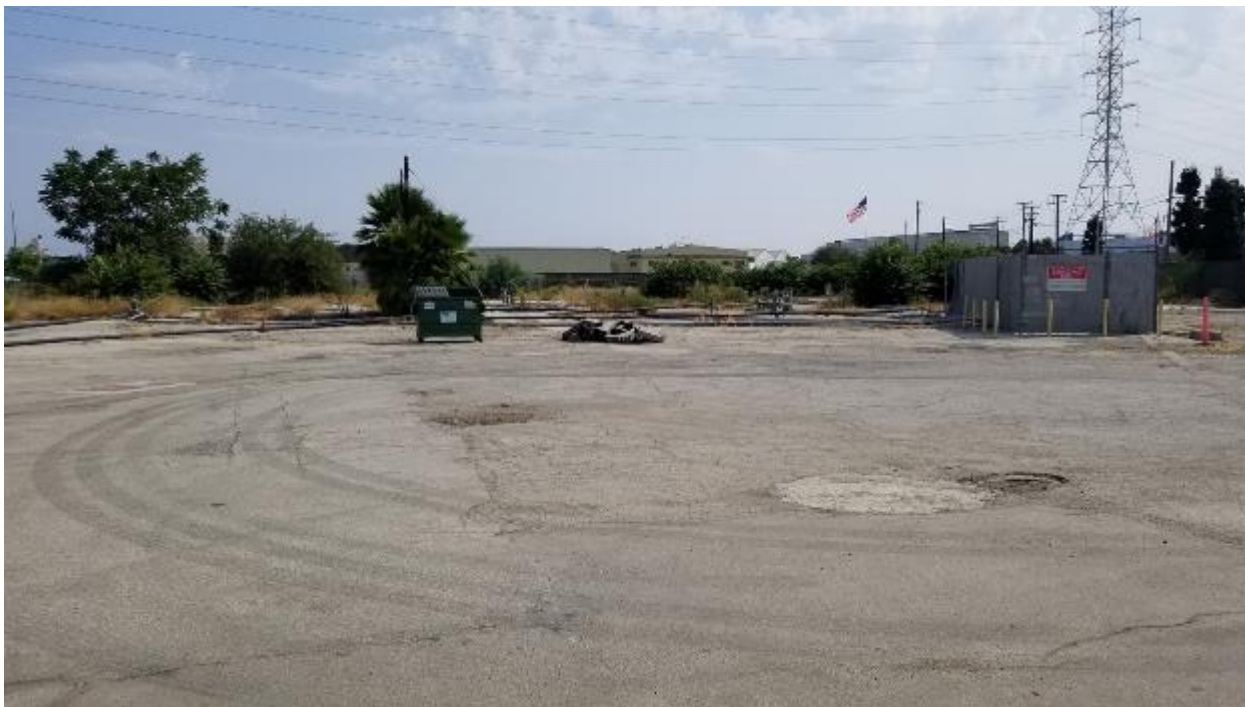
Figure 22. Overview of the well field. Facing north.
