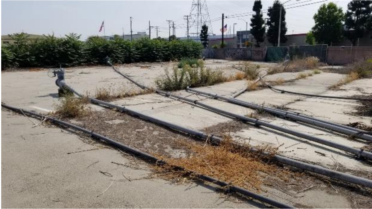
Figure 26. SVE lines. Facing northeast.
