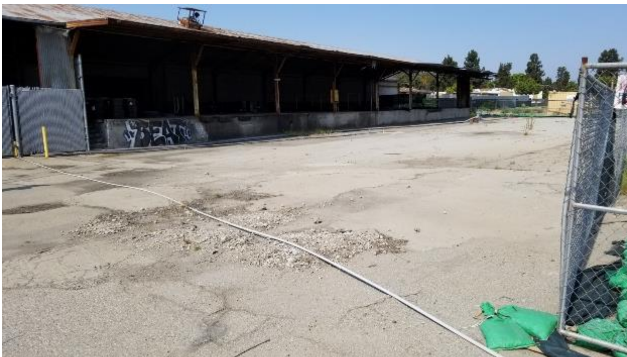
Figure 14. Drum Processing Area. Facing southwest.
