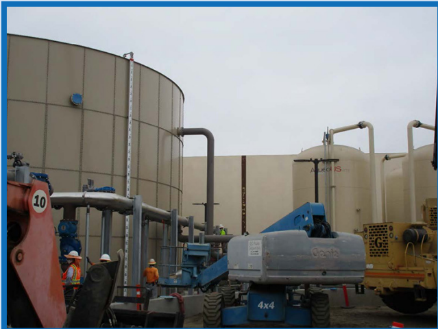
Construction of Puente Valley OU Intermediate Zone Treatment Facility, City of Industry.
