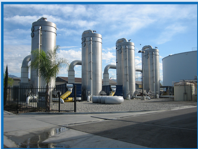
Groundwater Treatment System at One of Five Baldwin Park OU Treatment Systems.
