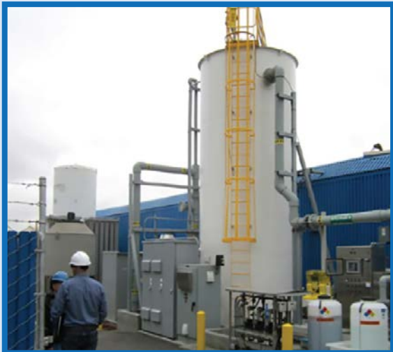
West Side Treatment System at El Monte OU.
