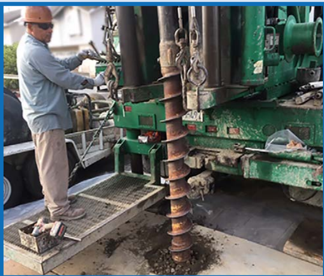
Drilling Monitoring Wells at South El Monte OU.
