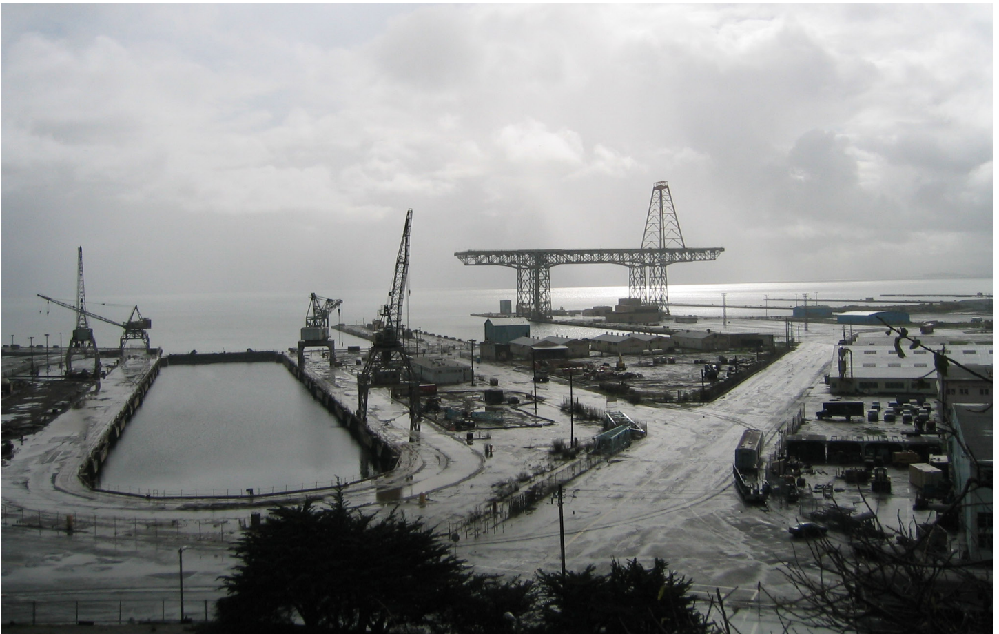
Historical photo of dry dock and gantry crane at the Hunters Point Naval Shipyard from the Naval History and Heritage Command.
