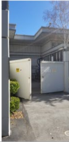
Siemens Remediation Compound
