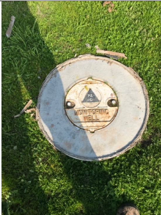
Monitoring well PZ-10
