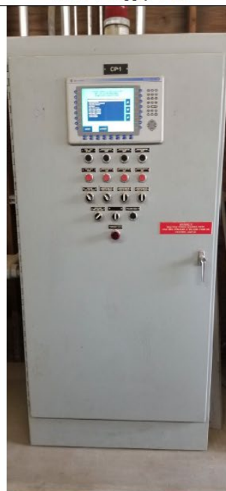
Rialto 3 Supply Well Control Panel
