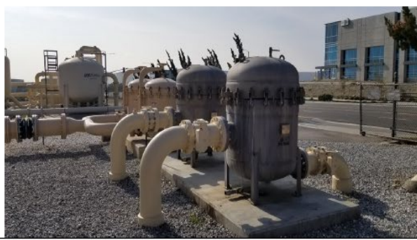
Rialto 3 Supply Well 5-Micron Bag Filters
