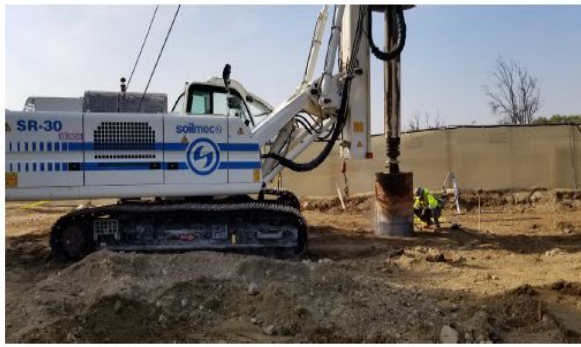
Drill Crews Installing 70-foot Dry Well at EW-1 Site
