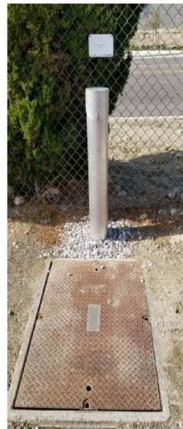
System Effluent Sampling Station & Signage
