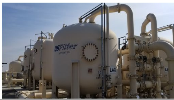
IX Resin Vessel (front) and GAC Vessels (rear)
