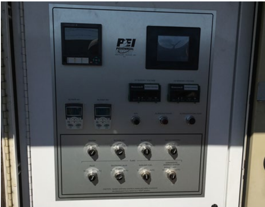
Photo 3 Cell A Flare control panel
