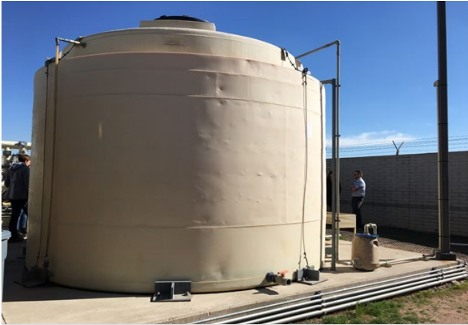
Photo 4 Cell A Flare condensation tank
