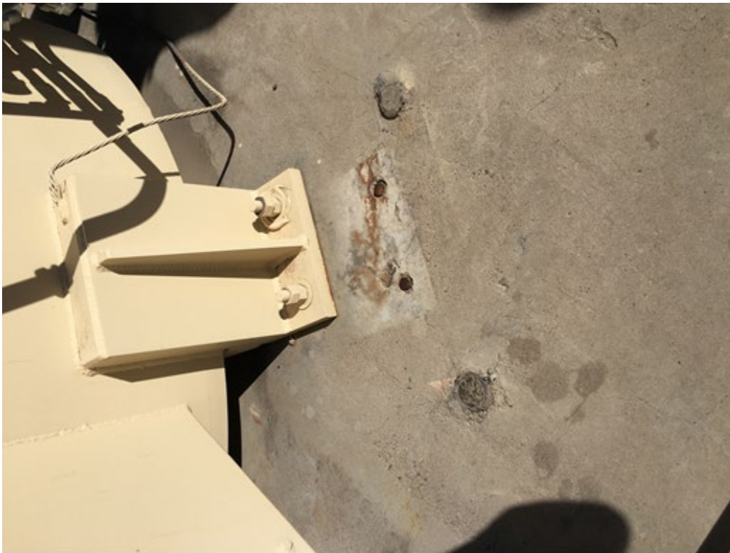
Photo 5 Flare stack mount, showing previous stack location
