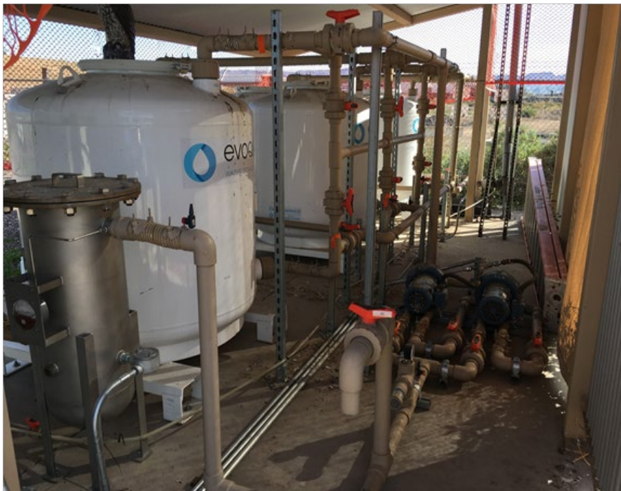
Photo 19 Cell A-1 GAC system
