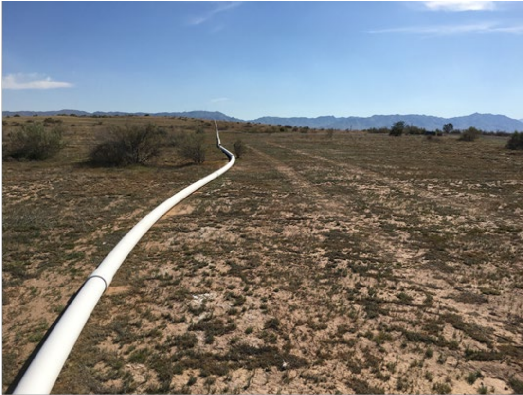
Photo 6 Overview of landfill cap, showing C-line of methane extraction system, facing south
