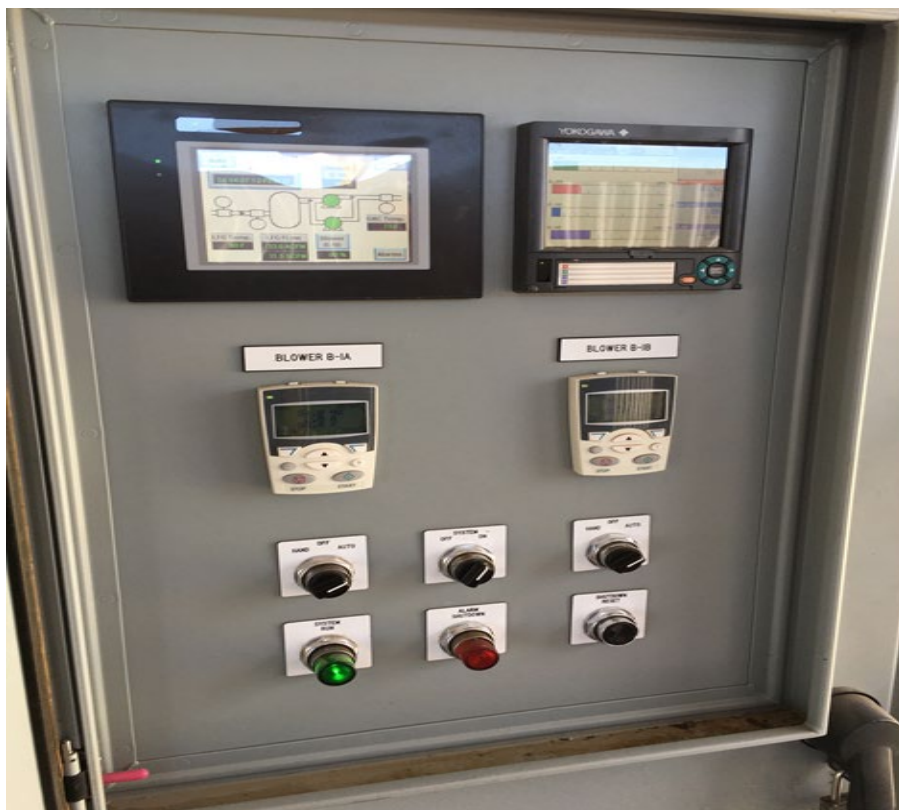
Photo 20 Cell A-1 GAC system control panel
