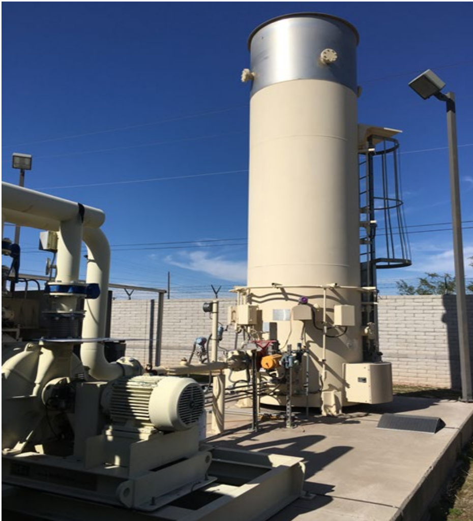
Photo 1 Cell A flare and blower
