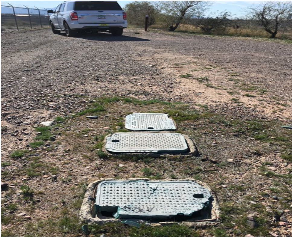
Photo 10 Gas collection well vaults in levee
