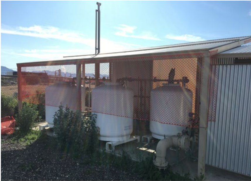
Photo 18 Cell A-1 GAC system
