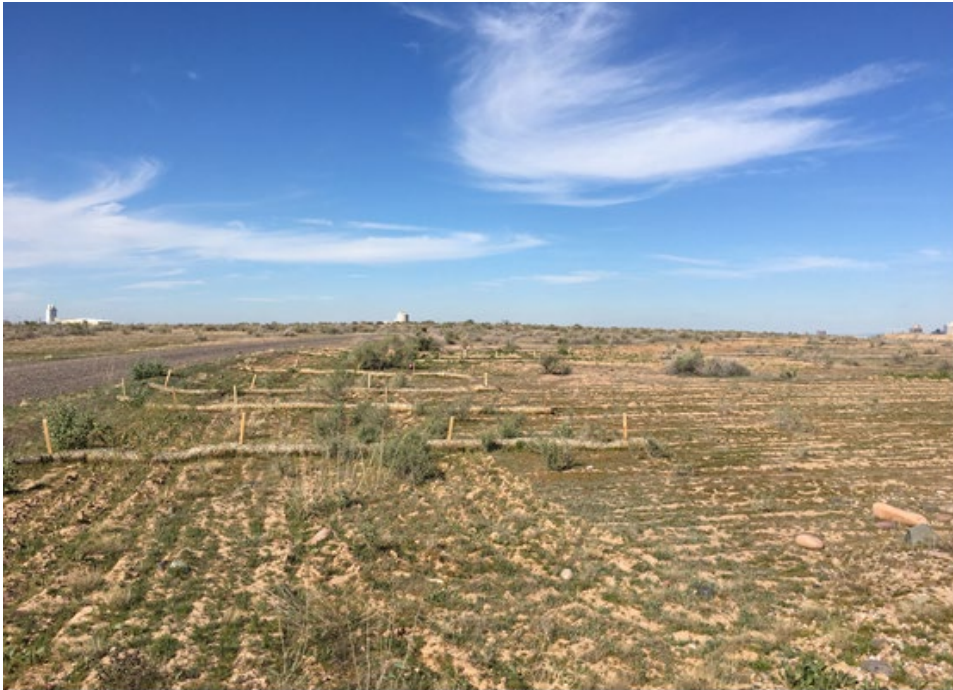
Photo 8 Straw wattles in place on cap, looking north
