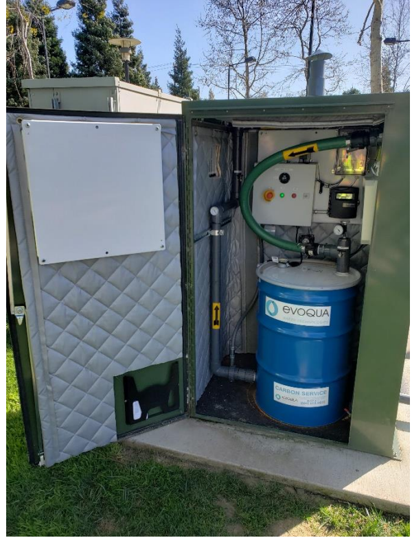
Vapor Intrusion Control System Carbon Treatment Unit – Raytheon – 350-380 Ellis Street
