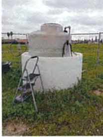
Examples of LC-1 and LC-3 tanks are displayed, where leachate collection is stored until sent off site as waste.
