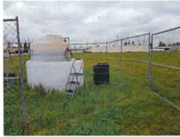
Examples of LC-1 and LC-3 tanks are displayed, where leachate collection is stored until sent off site as waste.
