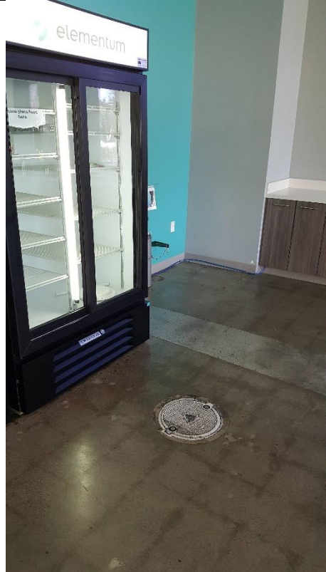
1300 Terra Bella Interior ERD Injection Well
