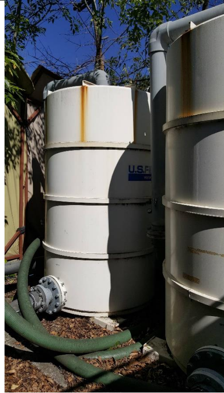
1300 Terra Bella Methane Mitigation System GAC Vessels
