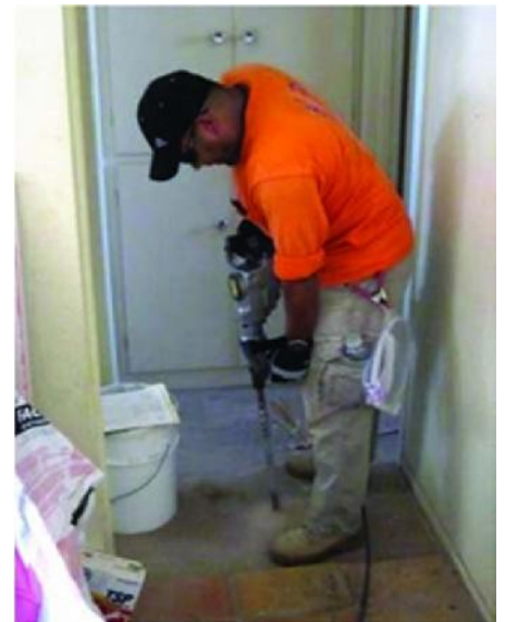
Sampling vapor under the slab.
