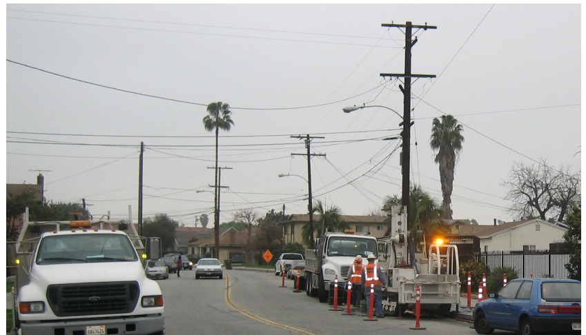
Construction activities at the SEMOU.
