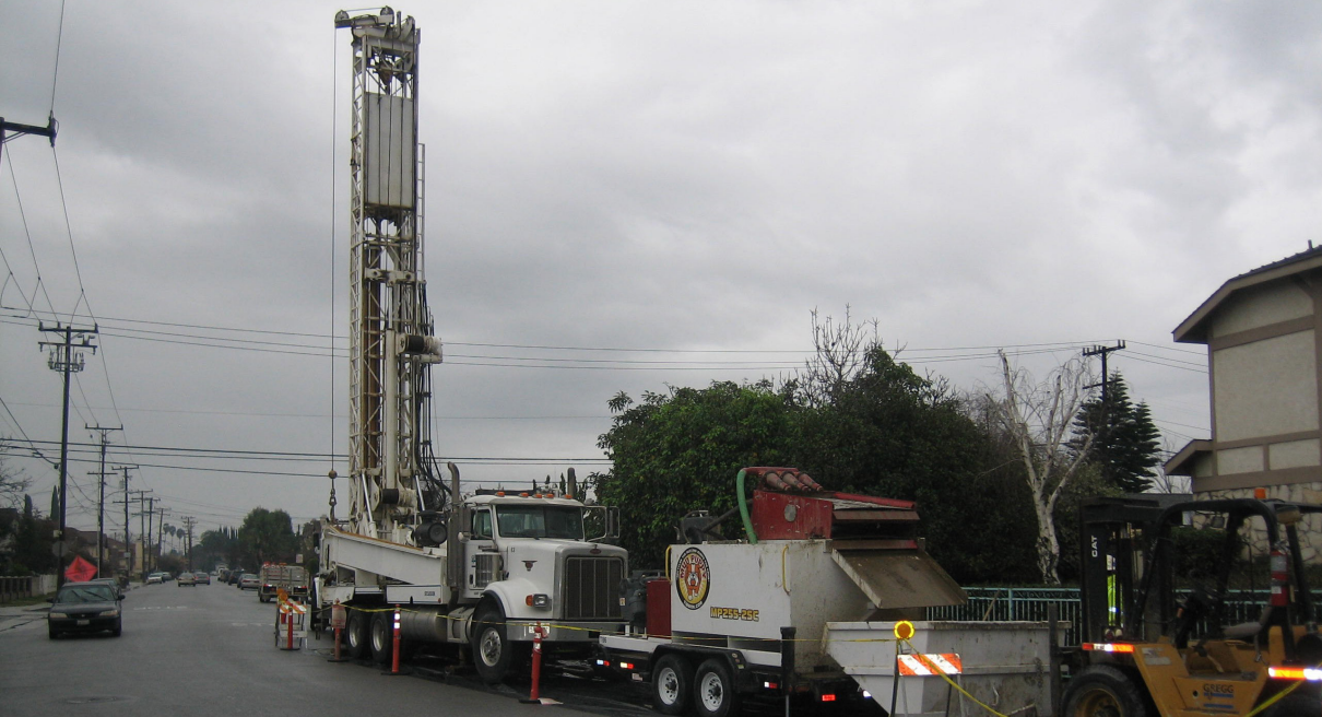
Well drilling at the South El Monte Operable Unit.
