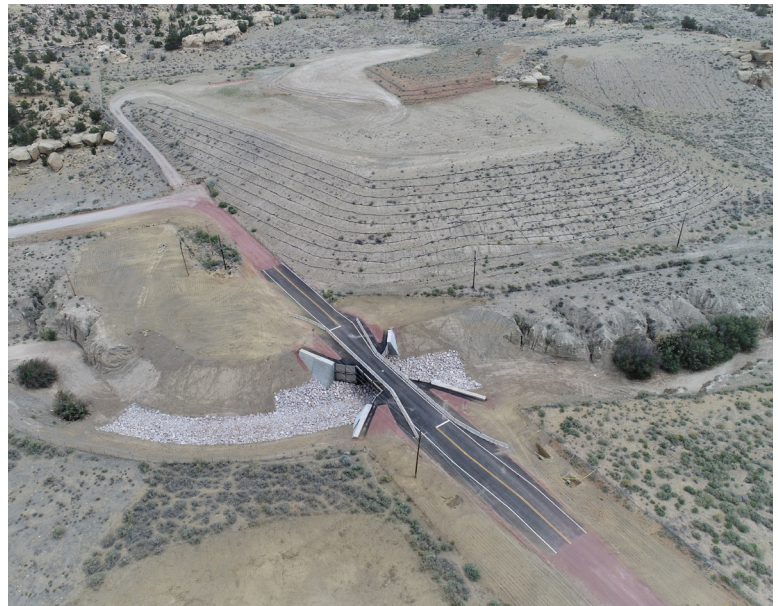
The Quivira mine waste pile and the newly repaired bridge.
