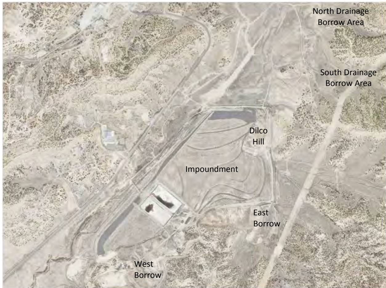
Figure 12. Cover Soil Borrow Areas
