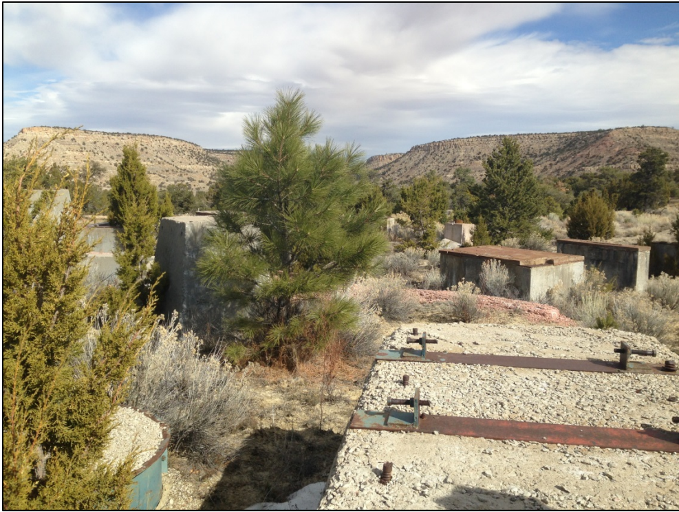
Photo C.4-1: Concrete Structures at Vent Hole Shaft Area
