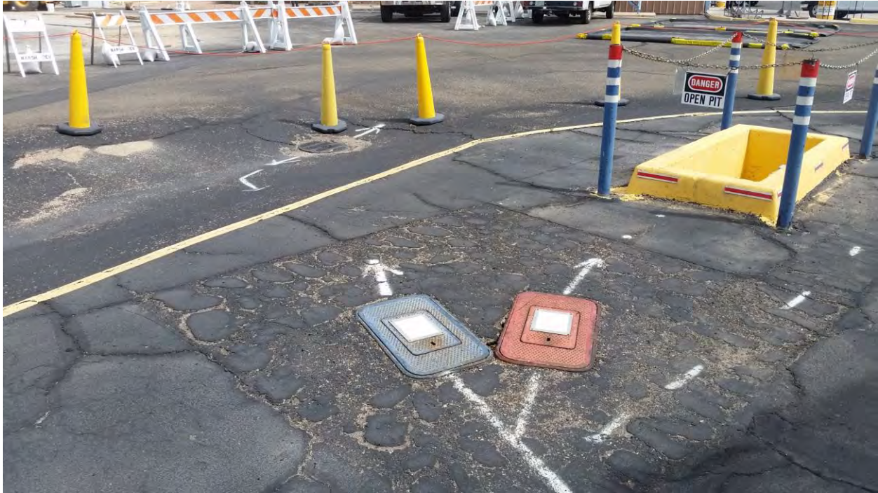
View to the Northeast of valve system at the wash rack; controls storm water runoff to storm drains versus aircraft wash water to the wash rack pretreatment unit prior to discharge to storm drain.
