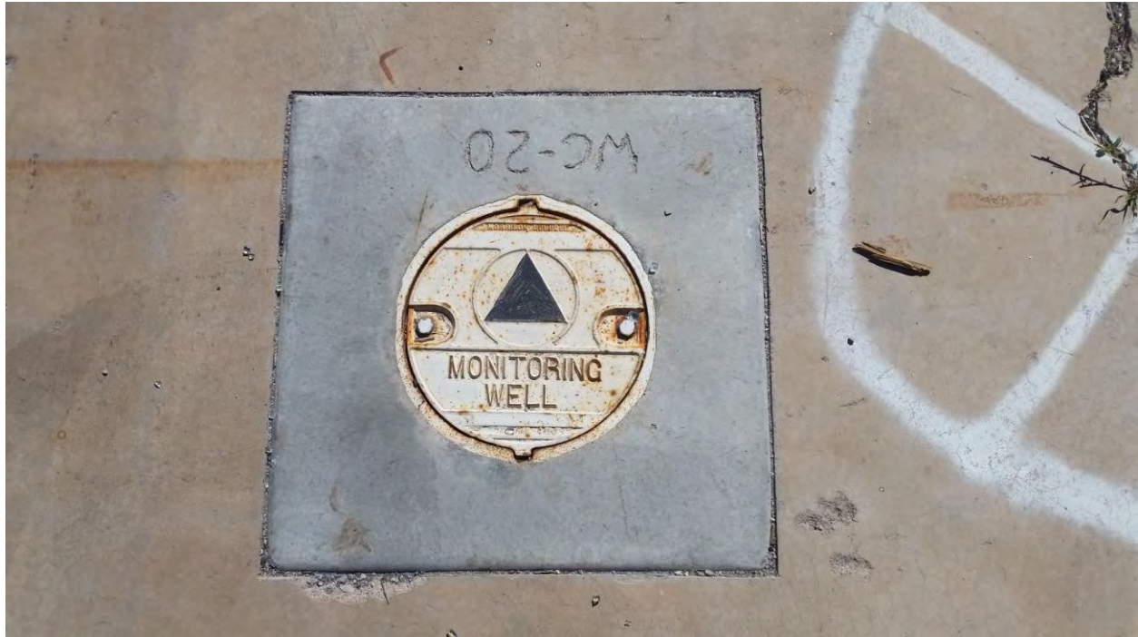
Typical nested injection and monitoring well at north end of concrete pad at Source Area.
