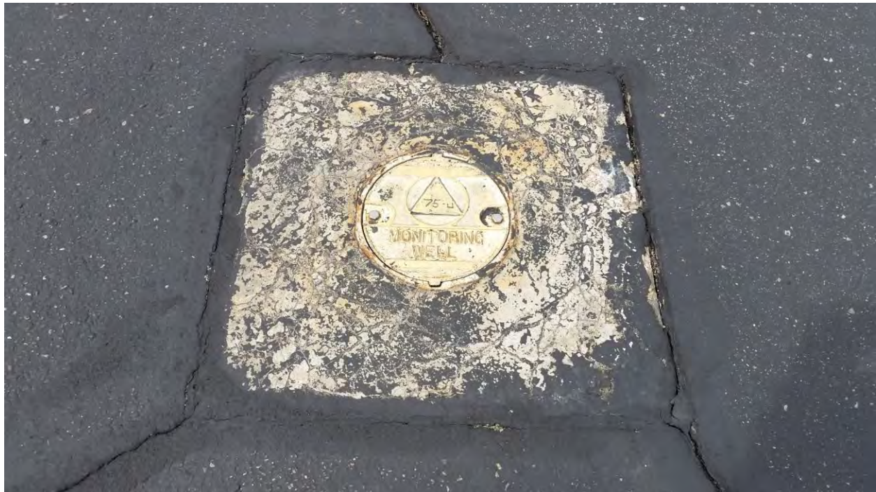
MW-75U typical monitoring well on AANG property.
