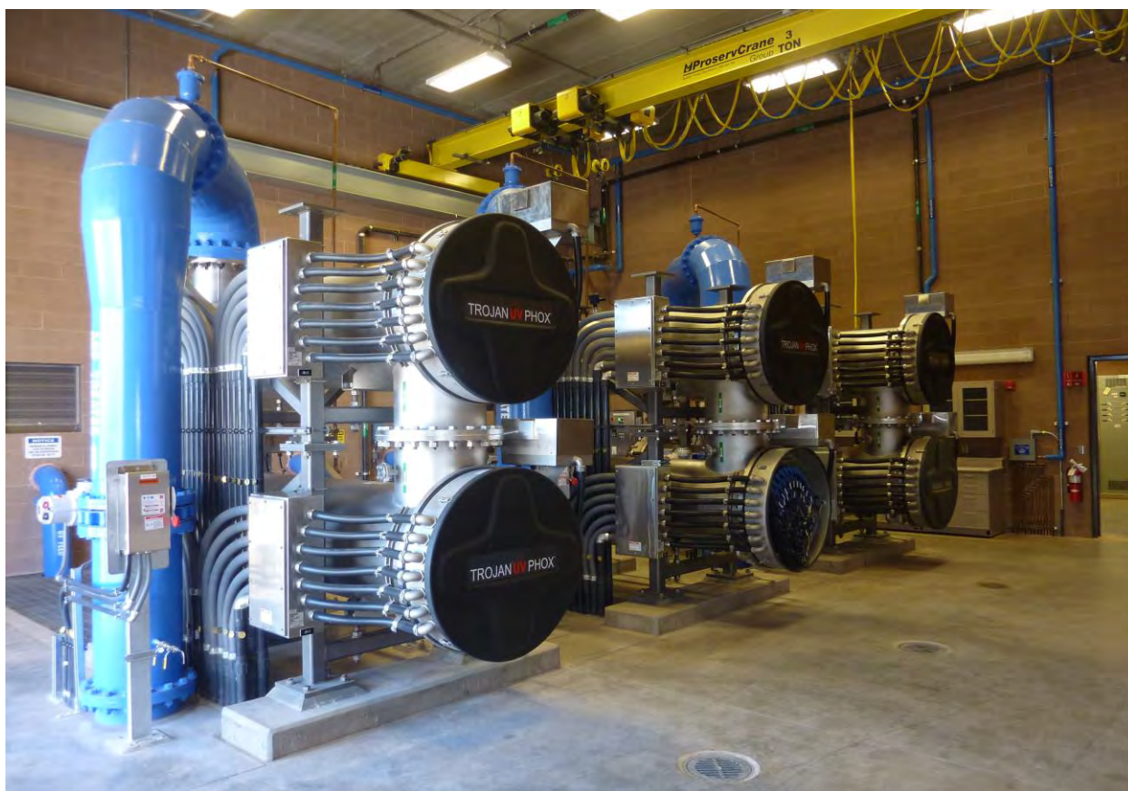
TARP AOP reactor trains.
