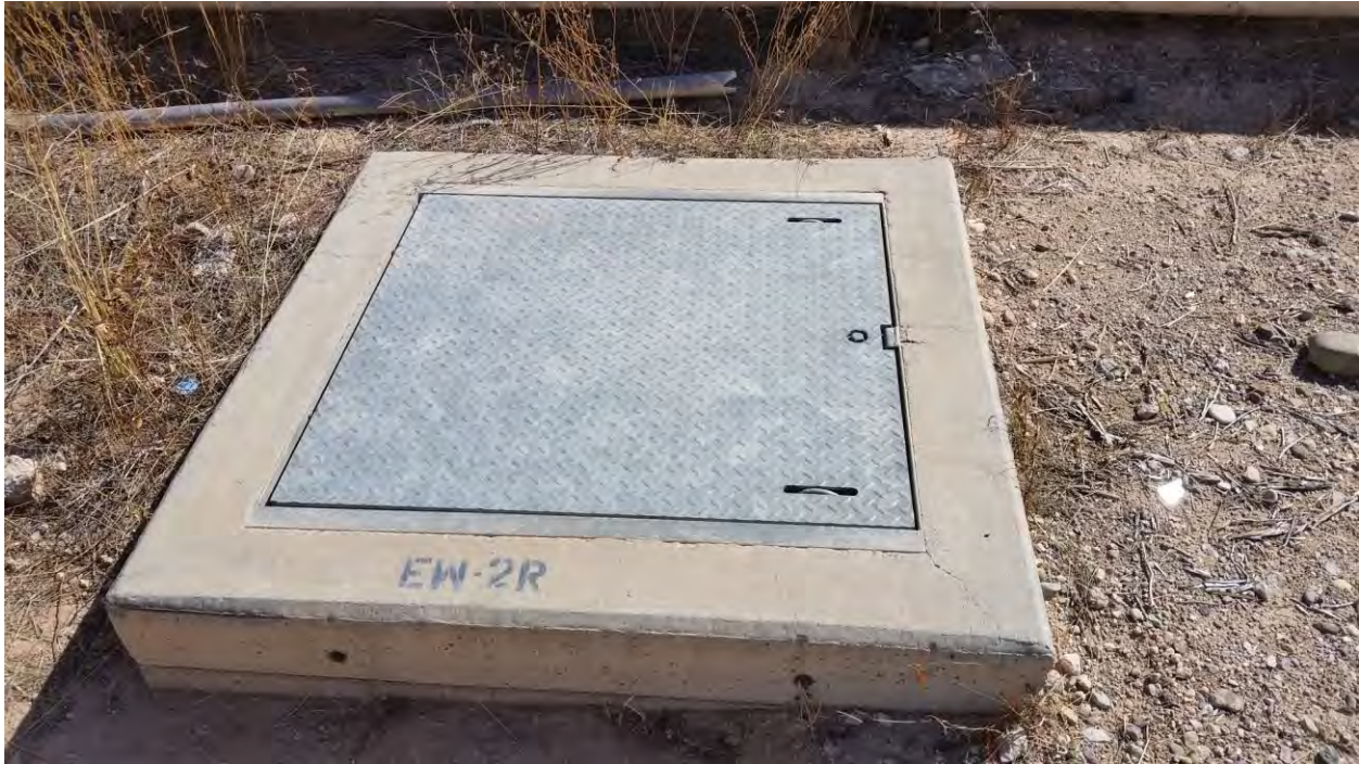
EW-2R groundwater extraction well.
