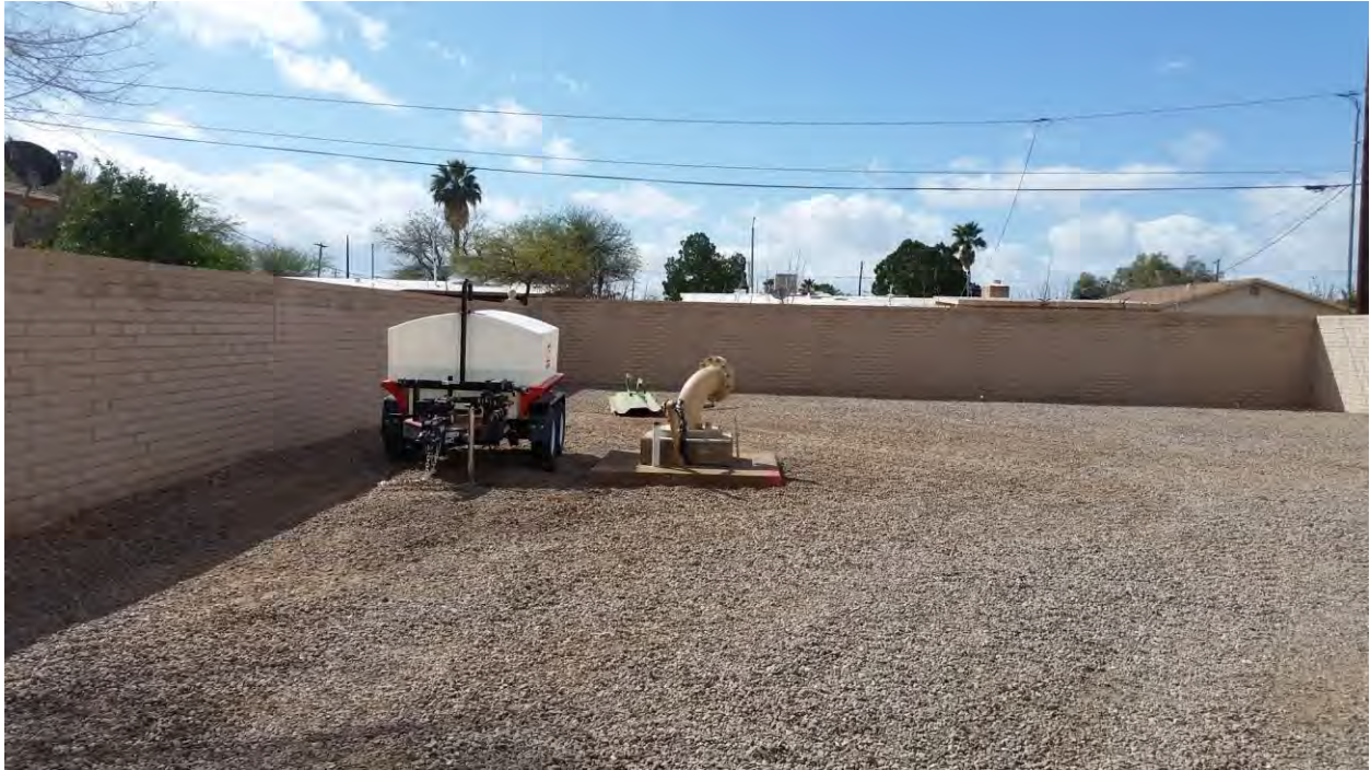
View to the South of remediation well R-008A; well taken out of service and surface piping removed in preparation for replacing the well with R-008B (due to poor condition of the well).
