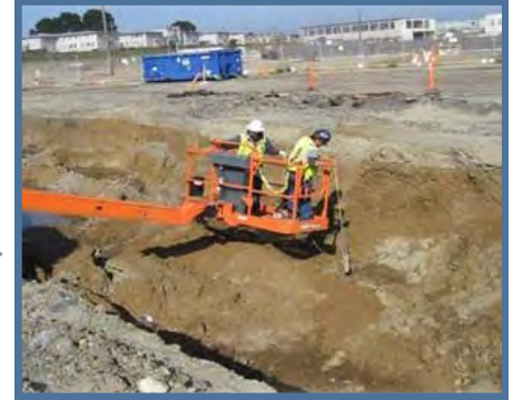
Radiological scans of trench sidewalls and floors may be conducted in-place
