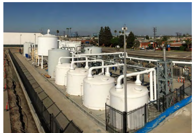
Groundwater treatment facility near Normandie Avenue on the Montrose property.
