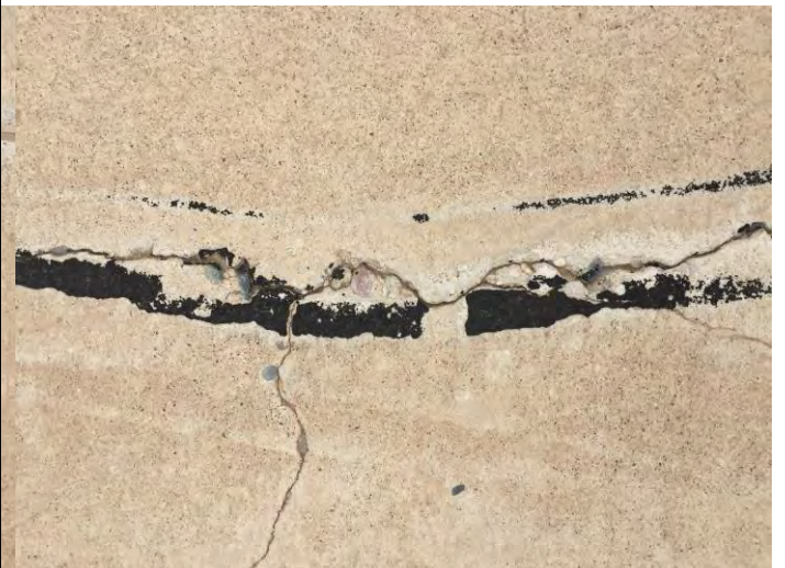
PHOTOGRAPH 30 – Site ST-18: Crack in concrete cap near center portion of site (view to west)
