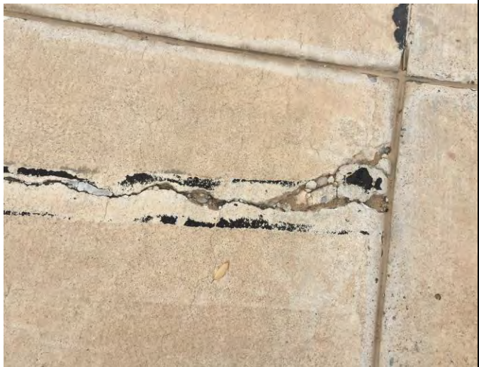
PHOTOGRAPH 29 – Site ST-18: Concrete cap showing previous tar/asphaltic sealant repair of cracks (view to west)
