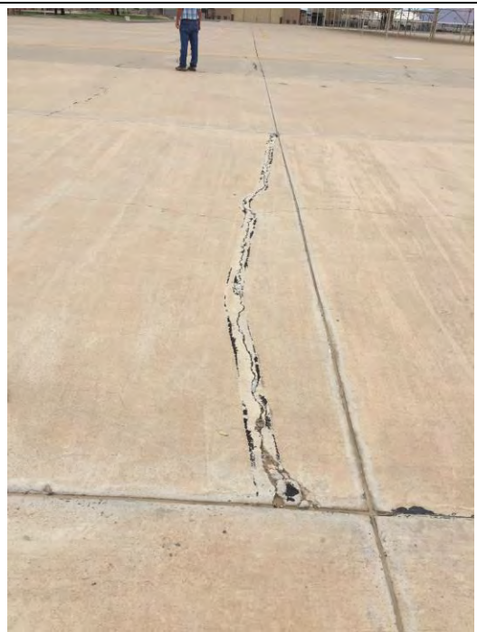
PHOTOGRAPH 30 – Site ST-18: Crack in concrete cap near center portion of site (view to west)
