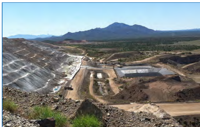
The Cyprus Tohono Mine Site, near the North Komelik community.
