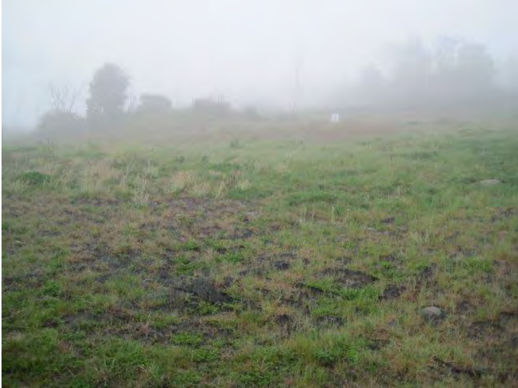
Photograph 17. Hillside at IR-18 at the southwestern corner of the cover looking southeast. Black is turf reinforcement matting that is not yet completely vegetated.
