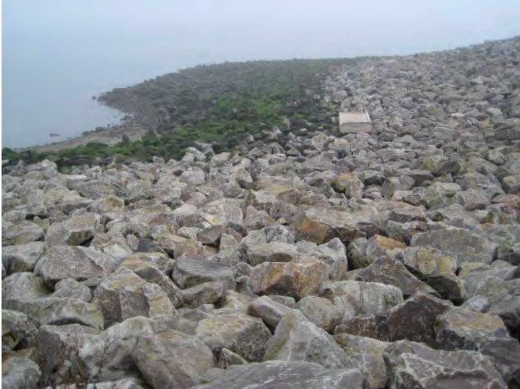
Photograph 7. Revetment looking east from central portion.
