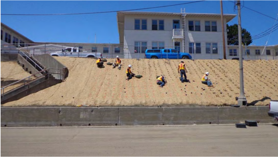
Planting newly covered hillslope with native plants
