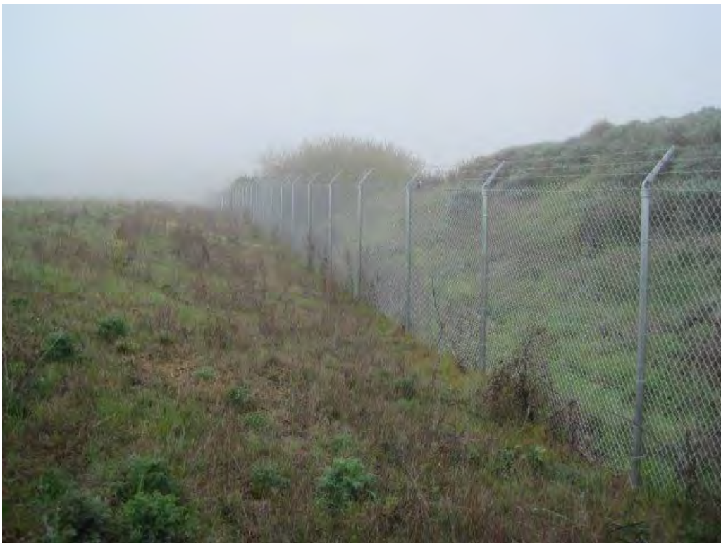
Photograph 12. Western boundary fence looking south. Cover side slope and vegetation.
