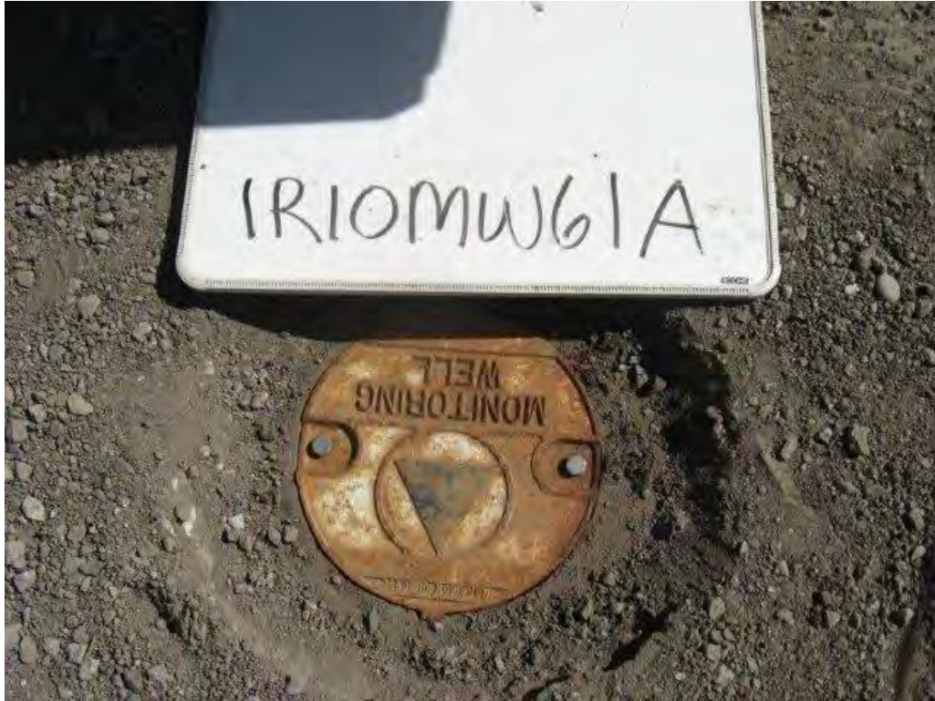
Photograph 57. Well IR10MW61A at Parcel B. Well box had been buried.
