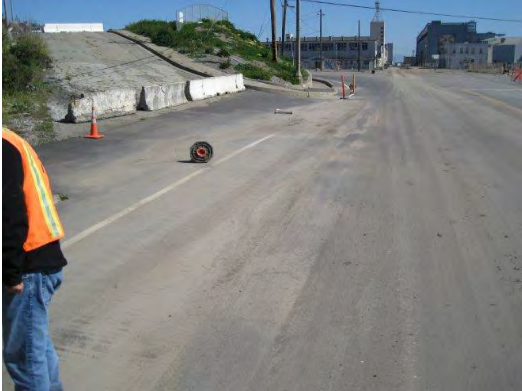
Photograph 43. Roadway at Parcel UC-1 (Spear Avenue) looking northeast. Lighter color on left is silt deposited from previous storm water ponding on the north side of the roadway.
