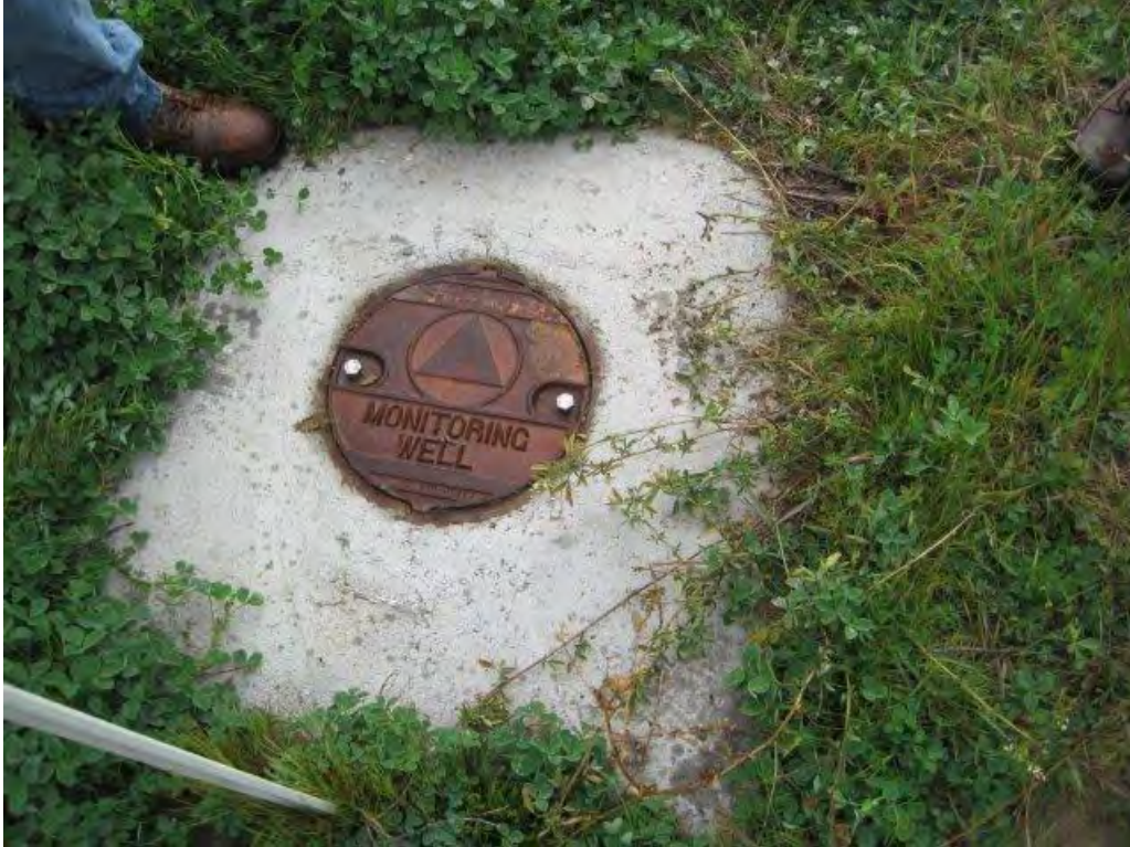
Photograph 29. Close-up view of well IR07MW24A.
