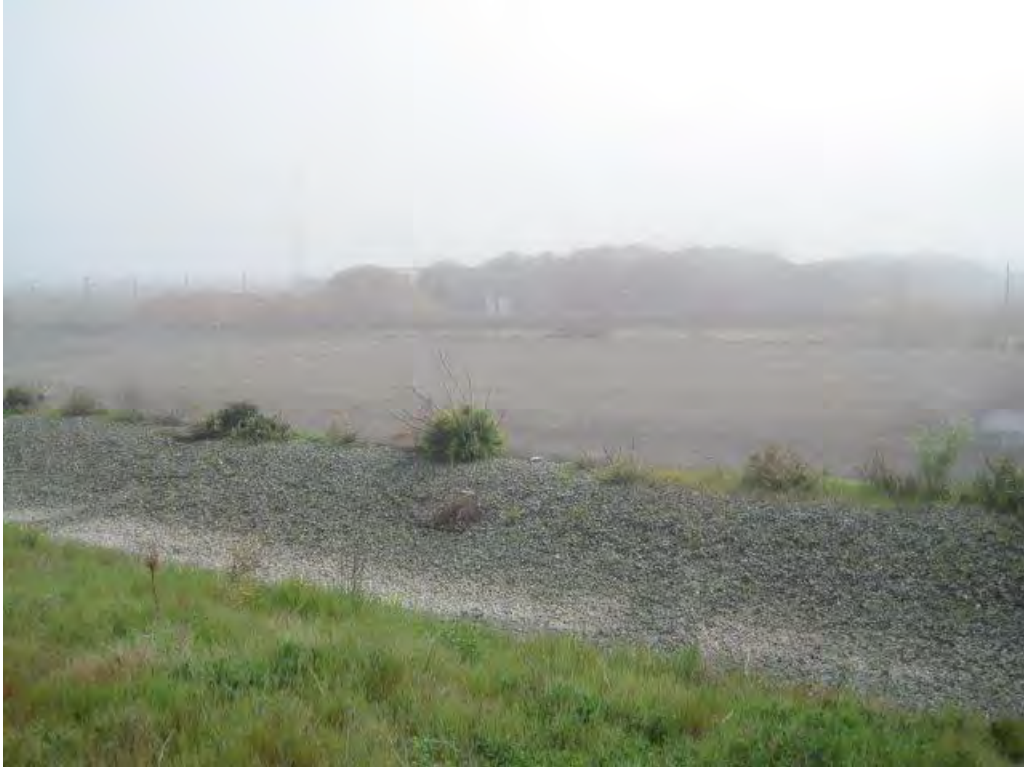
Photograph 25. Gravel-lined drainage swale in foreground. Asphalt cover over small portion of the northeastern part of IR-07 in the background. Looking east.
