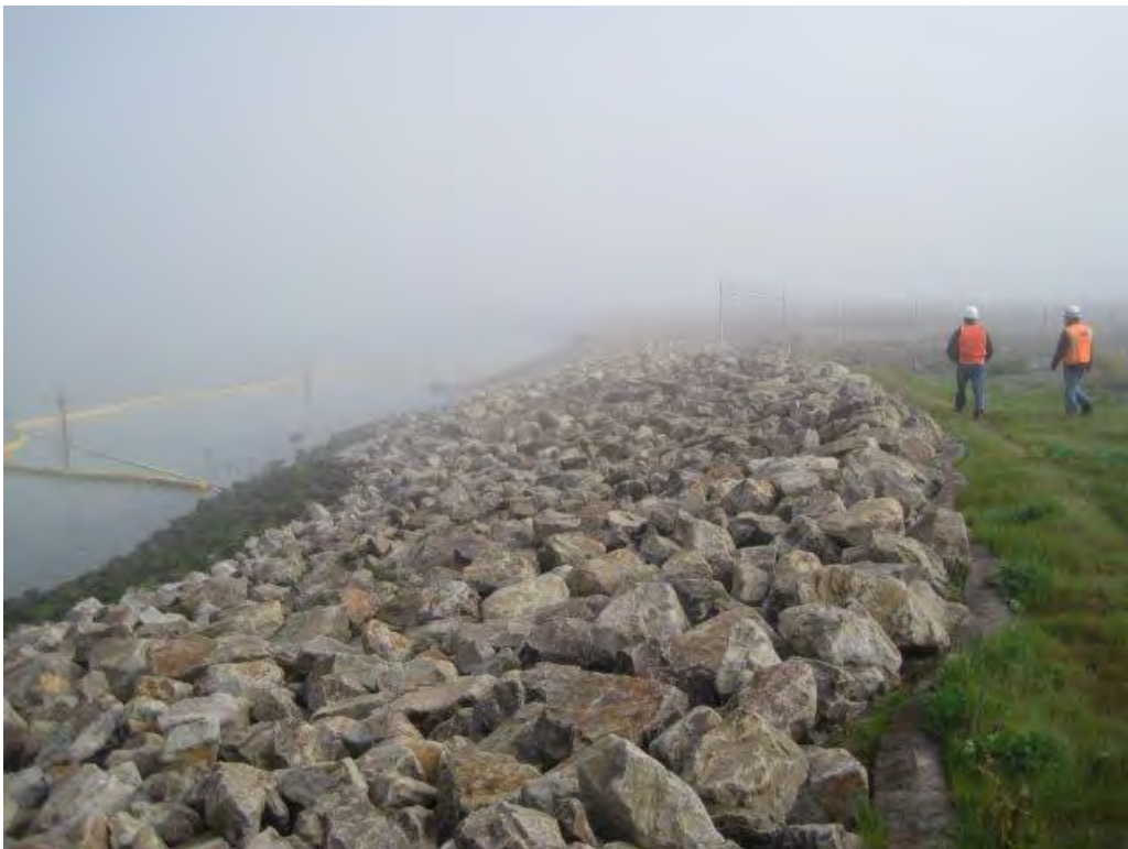
Photograph 26. Revetment tie in between IR-07 and IR-23, looking northeast.
