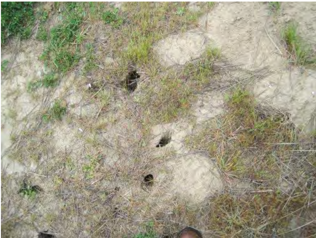
Photograph 14. Small burrows (1 to 2 inches in diameter) in the cover in the northwestern portion of the cover.
