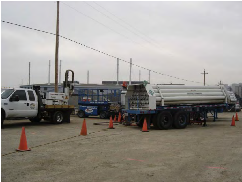
Injection of zero-valent iron to treat VOCs in groundwater
