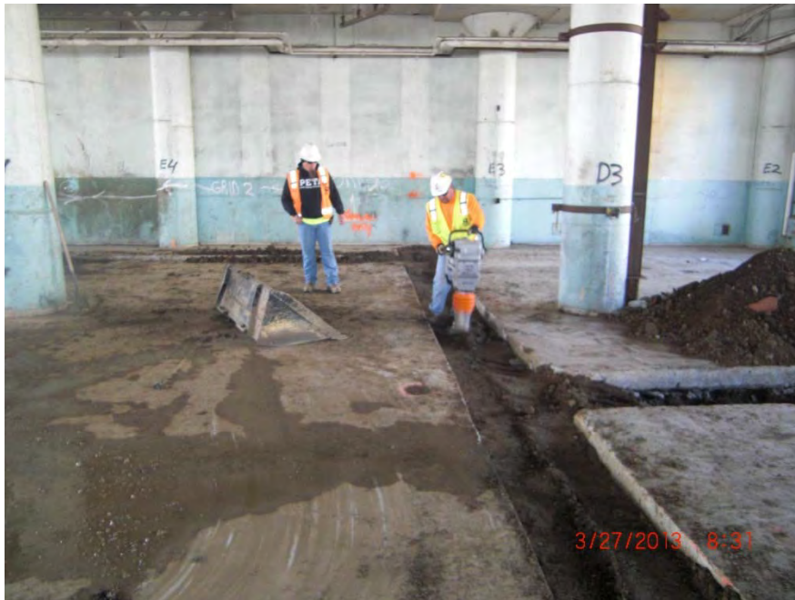
Repairing building foundations to act as covers
