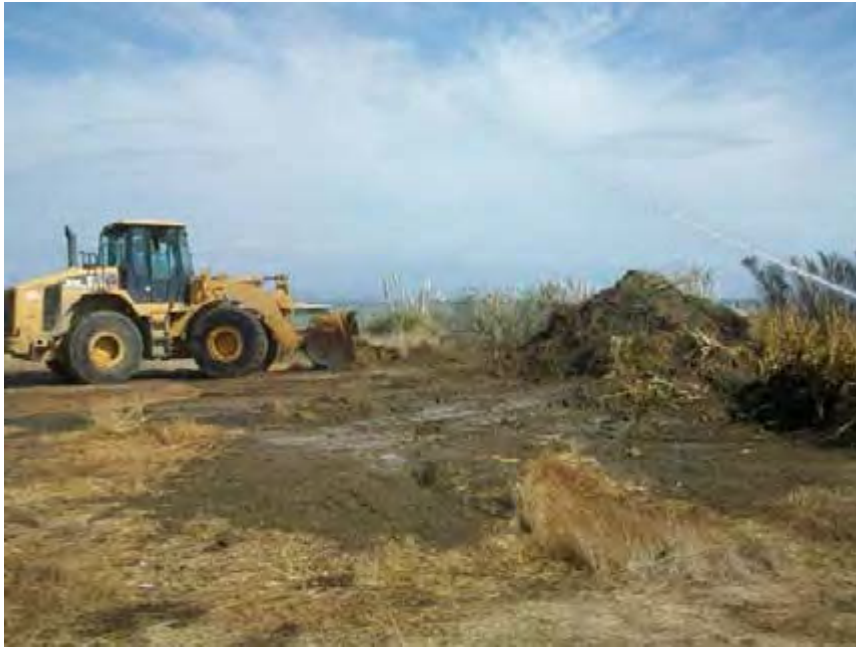
Excavation of hot spot soil areas and removal of soil stockpile
