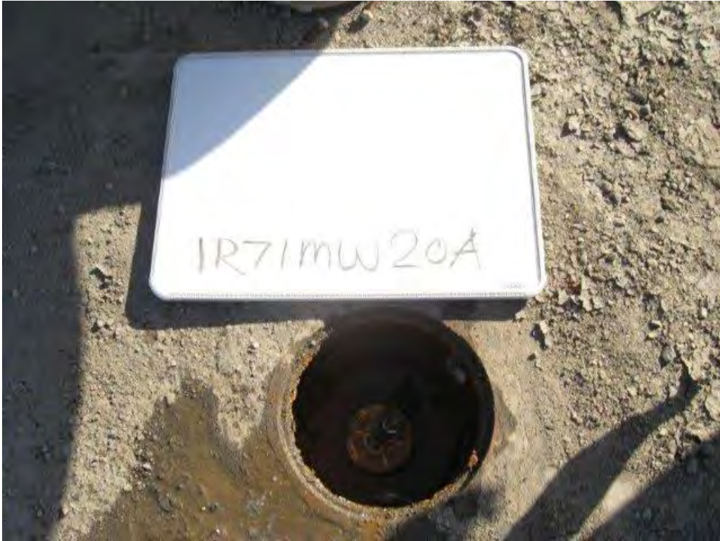
Photograph 67. Well IR71MW20A at Parcel D-1. Water inside well box.
