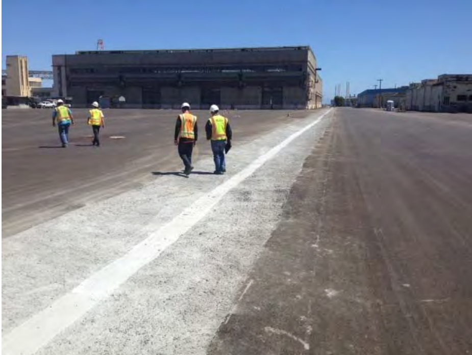
Completed paving and drainage swale at Parcel G
