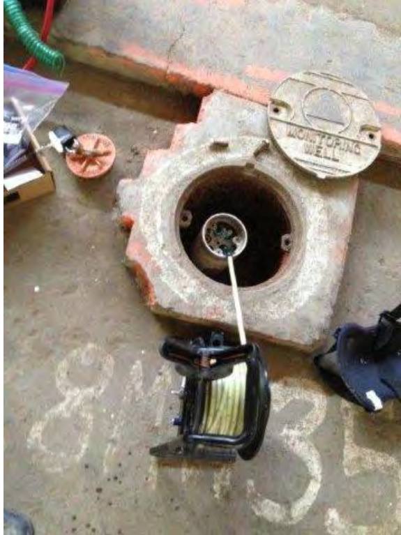
Photograph 63. Well IR28MW355F at Parcel C.
