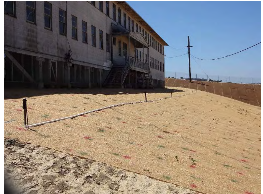
New 2-foot soil cover installed over slope; vegetation establishment in progress
