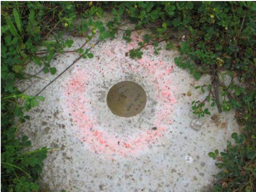
Photograph 6. Close-up view of cover settlement monument.
