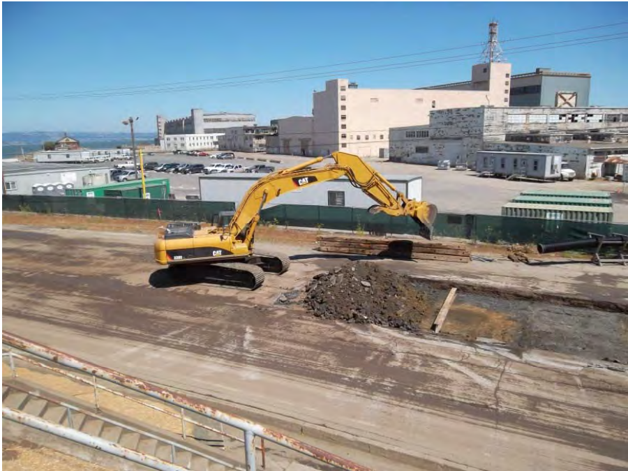
Asphalt pavement repair
