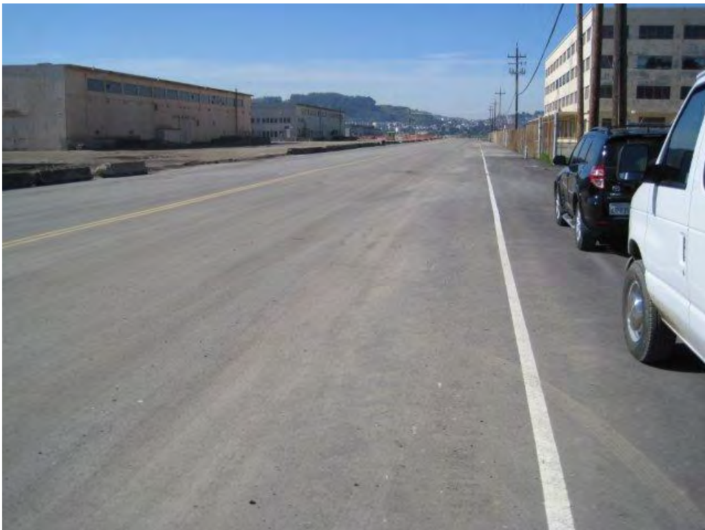
Photograph 42. Roadway at Parcel UC-1 (Spear Avenue) looking southwest.
