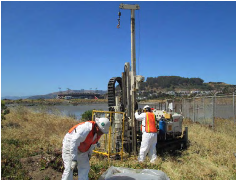
Installing soil gas monitoring probe
