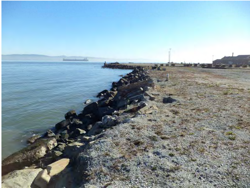
Original shoreline with concrete and metal debris
