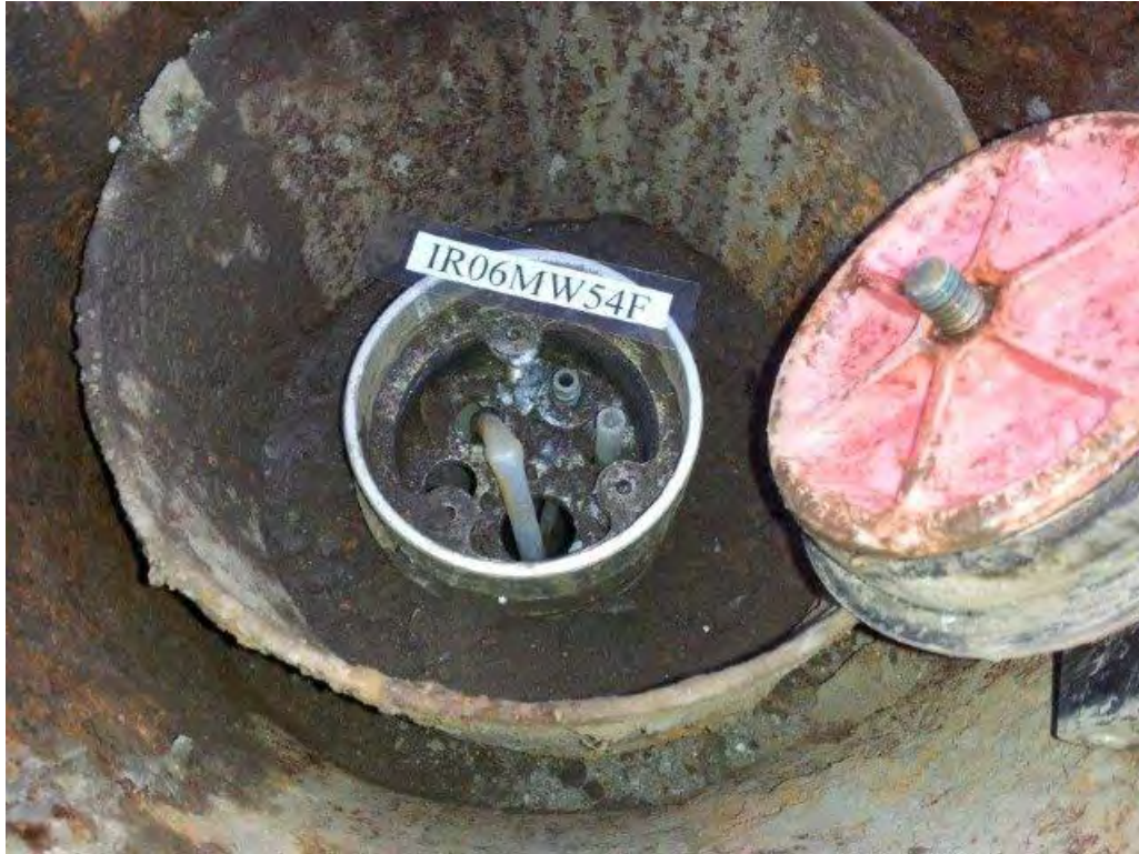
Photograph 49. Well IR06MW54F at Parcel UC-2.
