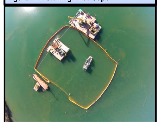
Figure 4: Installing Pilot Caps
