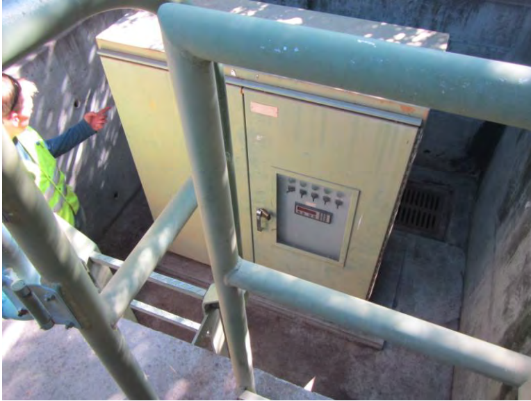
Photo 5. North Bayshore Extraction System control panel for E-8S
