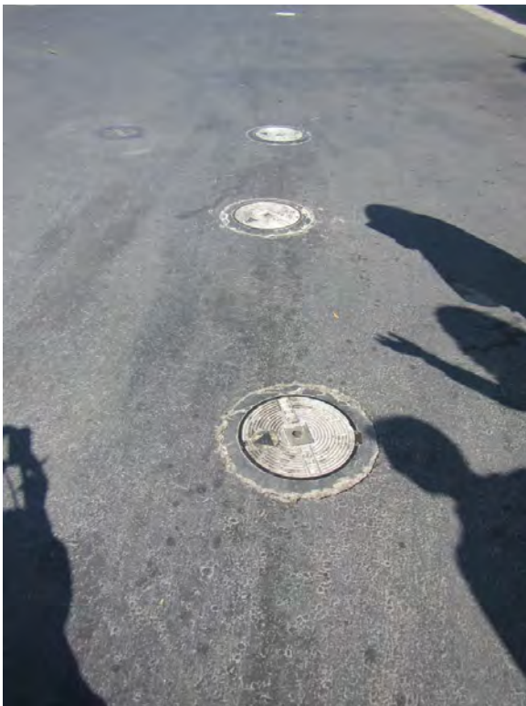
Photo 2. Enhanced bioremediation injection points
