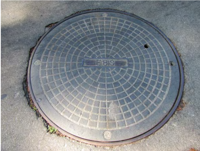
Photo 3. Extraction well E-8S
