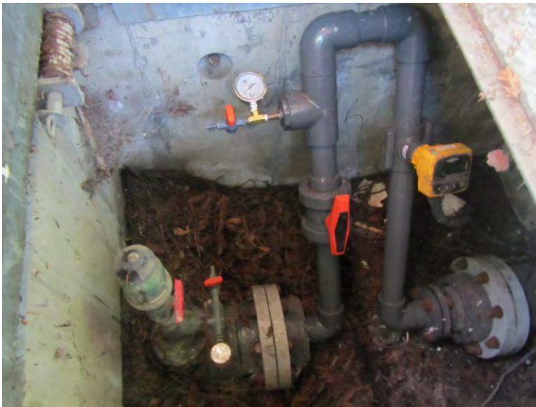
Photo 4. North Bayshore Extraction System sampling port
