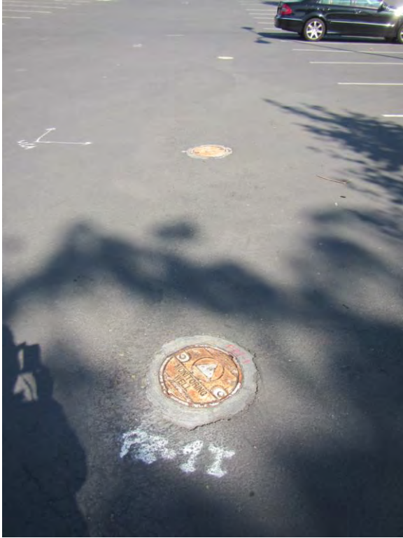
Photo 11. Typical monitoring well
