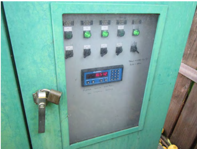
Photo 8. Control Panel for Spring Street Extraction System
