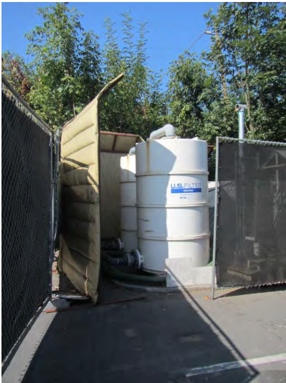
Photo 12. Methane SVE system with sound barriers
