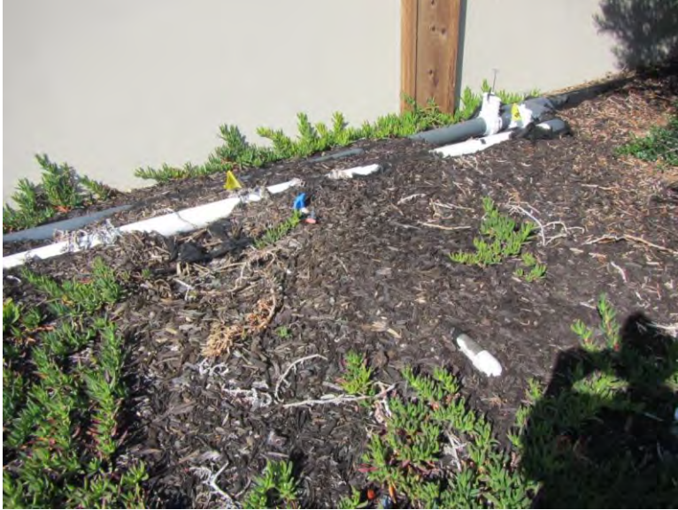
Photo 13. Methane extraction well and header
