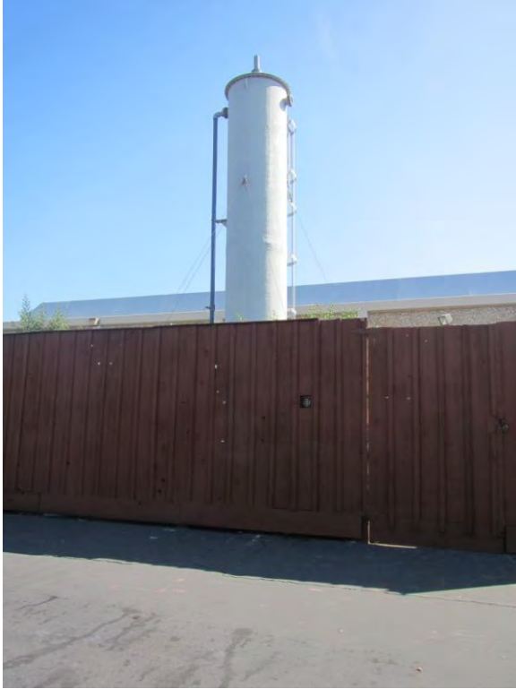
Photo 1. Air stripper (not in use)
