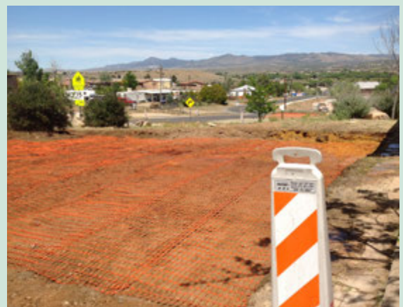
EPA placing a warning marker (or "snow fence")
