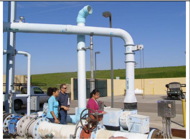
Packed tower bypass
