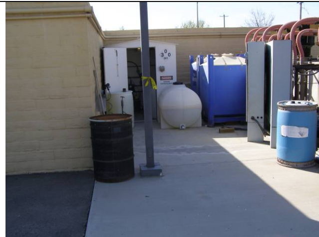
Chemical addition building
