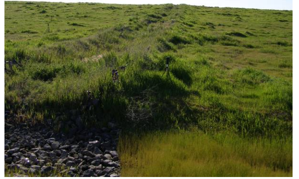
Drainage channel on slope of landfill
