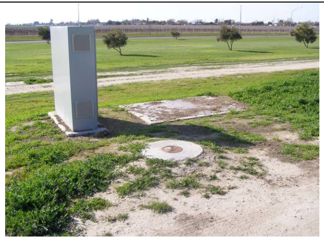
Groundwater extraction well and monitoring well
