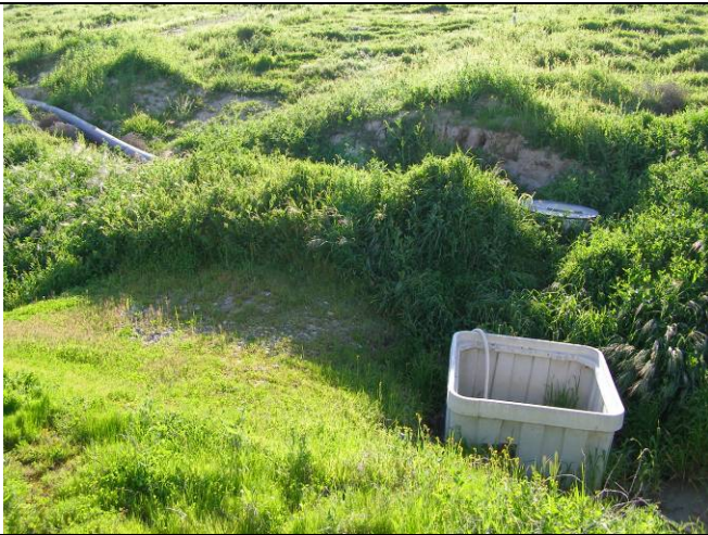
Gas condensate piping
