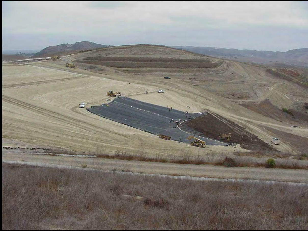
Installation of RCRA cap on metals landfill as part of early action work in 2002. Caustics/Cyanide Landfill appears in background.
