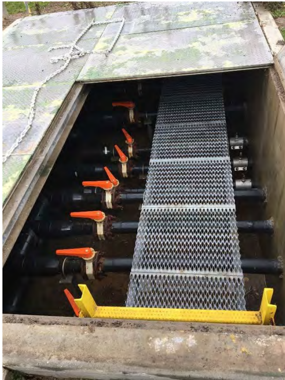
Photograph 8. Piping and valves for the GCTS for the Los Coyotes and Ramparts Sump areas. Catwalk installed for worker safety.
