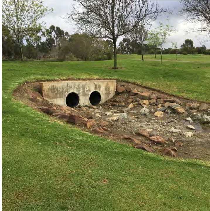
Photograph 10. Stormwater outlet from the retention pond. Outlet is armored with large rock and appears to be functioning as designed.
