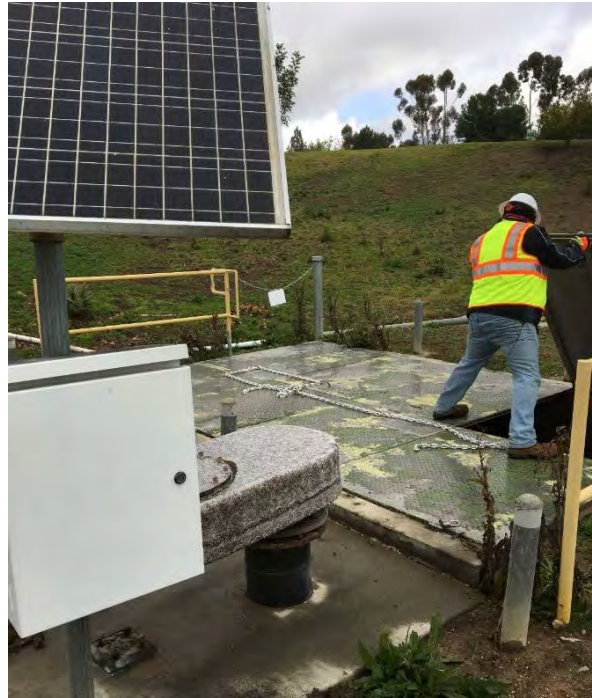
Photograph 7. Access hatch for the manifold for the Gas Collection Treatment System (GCTS) installed to manage vapor extending from the Los Coyotes and Ramparts Sumps.
