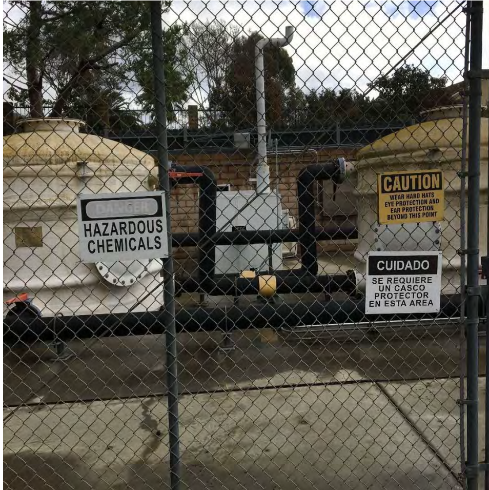
Photograph 12. Remediation enclosure with appropriate signage displayed on the fencing. Remediation enclosure is located in the northwest corner of the property near Rosencranz Avenue and Sunny Ridge Drive.
