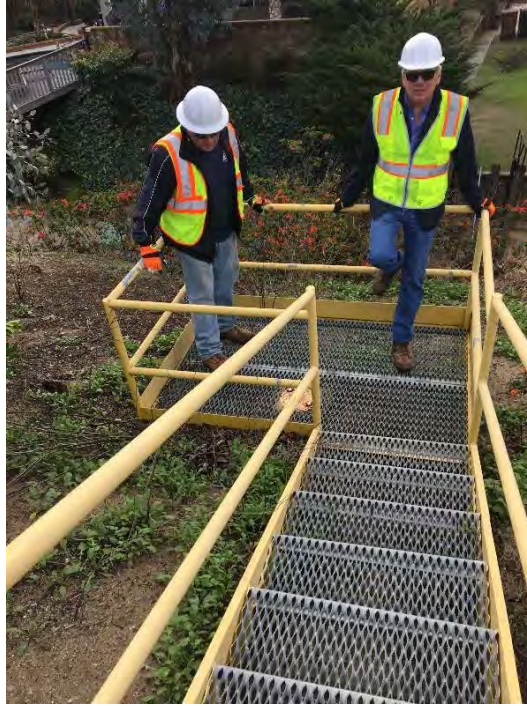
Photograph 5. Sampling platform installed for a well on the steep slope of the Ramparts Sump Area. Platform was installed to protect worker safety when sampling.
