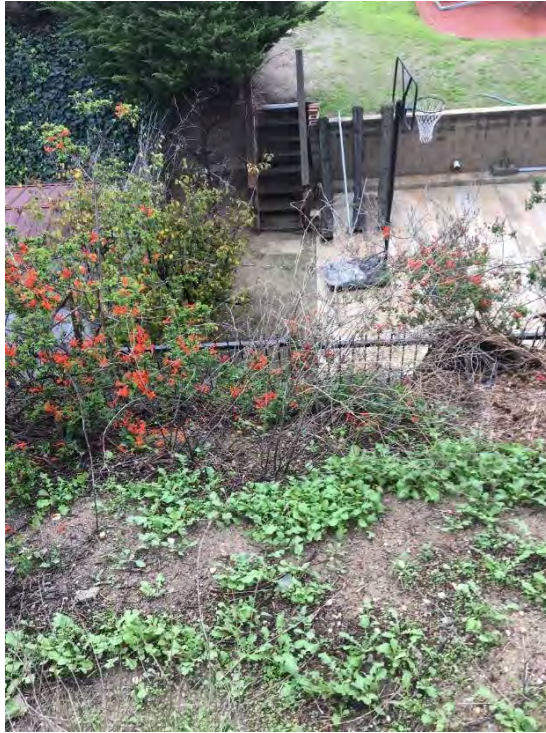
Photograph 4. Standing on the edge of the Ramparts cap looking downward to adjacent residential property. C2 REM indicates that the retaining walls are functioning as designed and no issues have been encountered since the 2012 five-year review.
