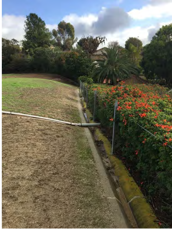
Photograph 2. Drainage ditch surrounding the Ramparts sumps.
