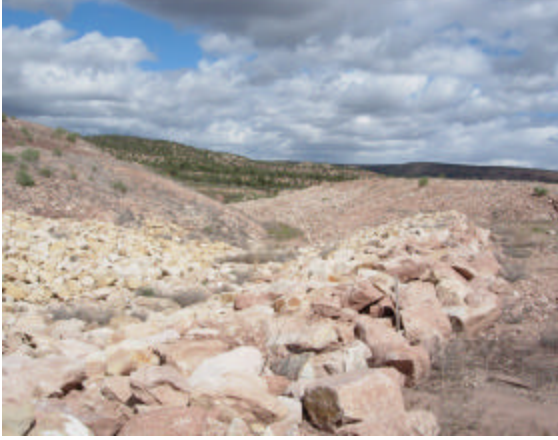
Club Mesa Tailings Pile 3 Storm Water Run-Off Control Feature
