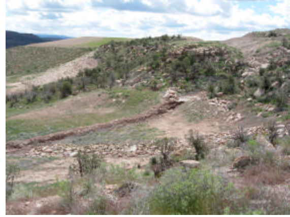
Club Mesa Storm Water Run-Off Erosion/Washout Feature
