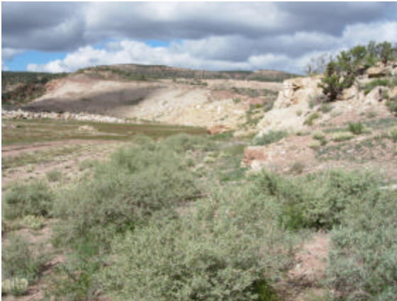
Photo of Tailings Pile 3 Repair of Suspected Joint Separation
