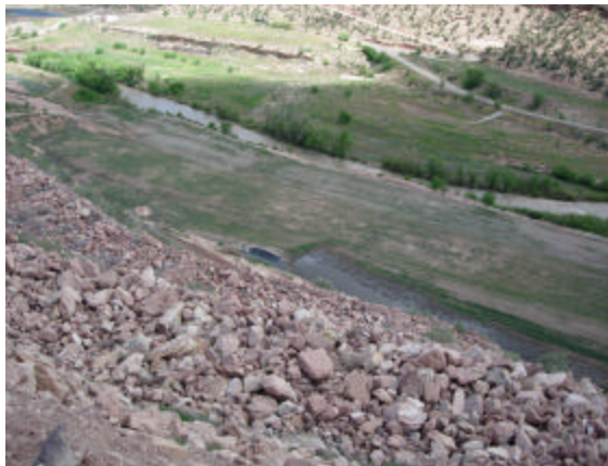
Hillside Area Seepage Collection Pond
