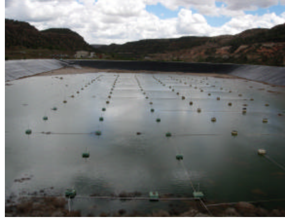
Club Ranch Pond CRP #8 Evaporative Spray system
