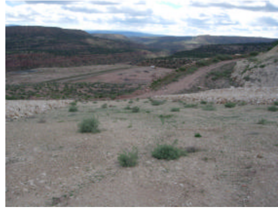
Club Mesa Tailings Pile 3 Partially Capped Repository
