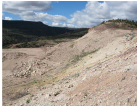
Photo 1 of 4 of Tailings Pile 3 Repair of Suspected Joint Separation
