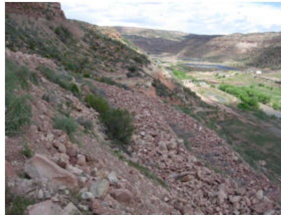
Reclaimed Mill Hillside Area with Storm Water Run-Off Erosion Control Features
