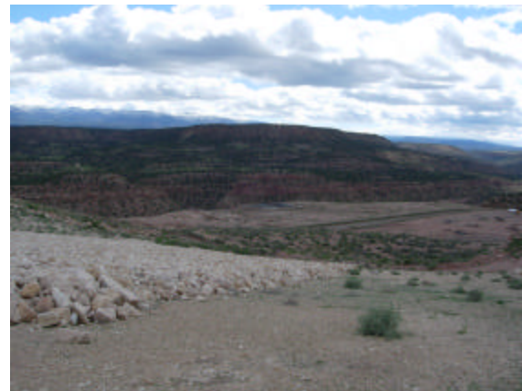
Club Mesa Tailings Pile 3 Partially Capped Repository
