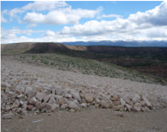
Club Mesa Tailings Pile 1 & 2 Partially Capped Repository
