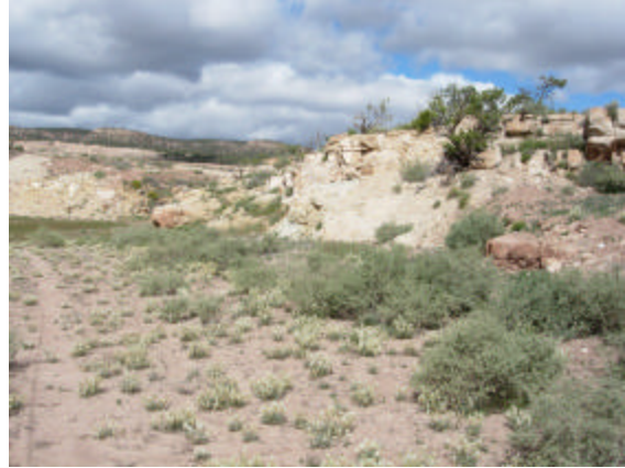
Photo 3 of 4 of Tailings Pile 3 Repair of Suspected Joint Separation
