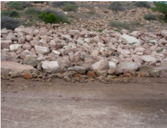
Hillside Area Seepage Collection Channel
