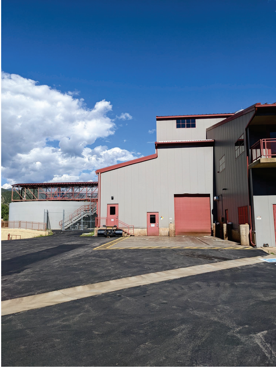
Argo Tunnel Water Treatment Plant
