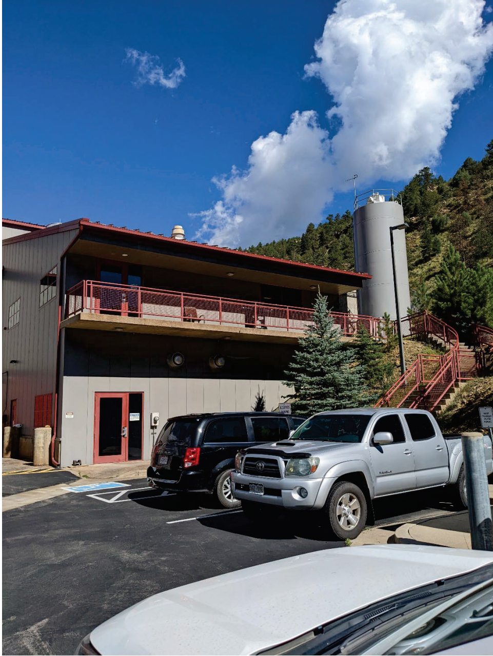
Argo Tunnel Water Treatment Plant
