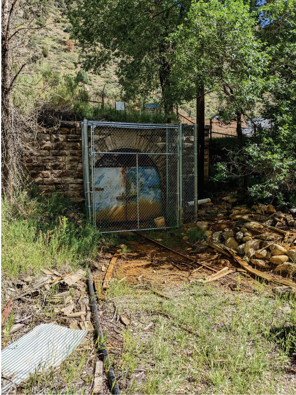
Big Five Tunnel Portal
