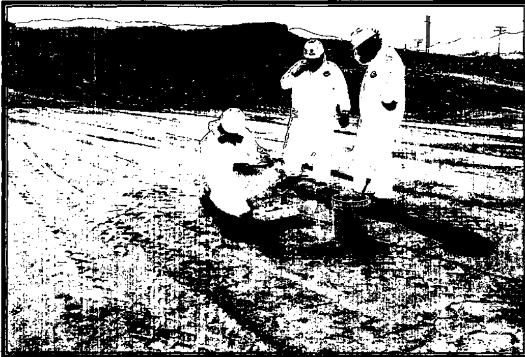
Photo 21: Consolidation Area —Looking East (June 19, 2003—During Field Compaction Testing of Initial Lift of Impacted Material)
