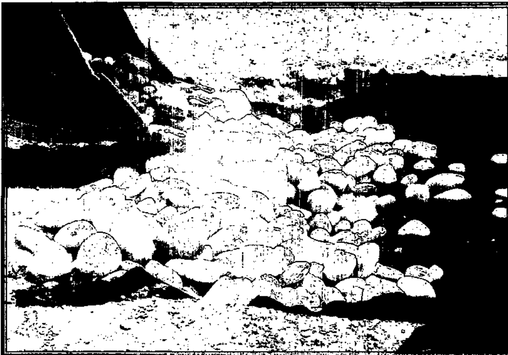
Photo 20: Discharge Apron—Looking East (August 7, 2003—During Placement of 6-Inch D50 Rock Riprap Material)
