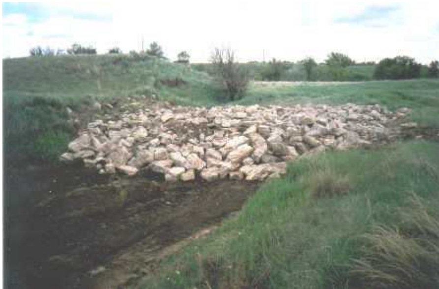
May 2001. Rip-rap at north end of soil disposal cell after placing Whitewood Creek Soil Samples inside cell. Photo taken looking south/southeast.
