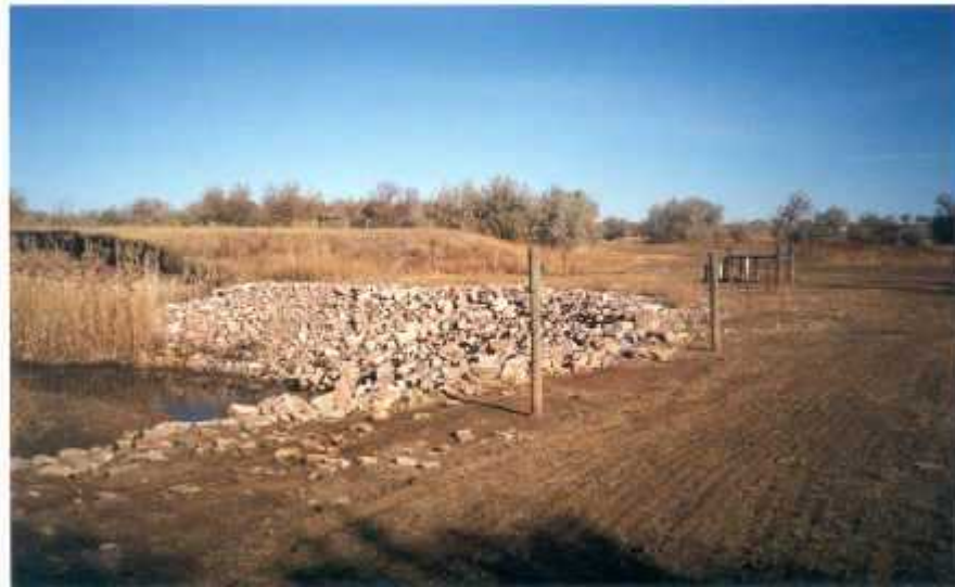
October 2000. View of rip-rap bank stabilization area and reseeded area. Photo taken looking to the north/northwest.
