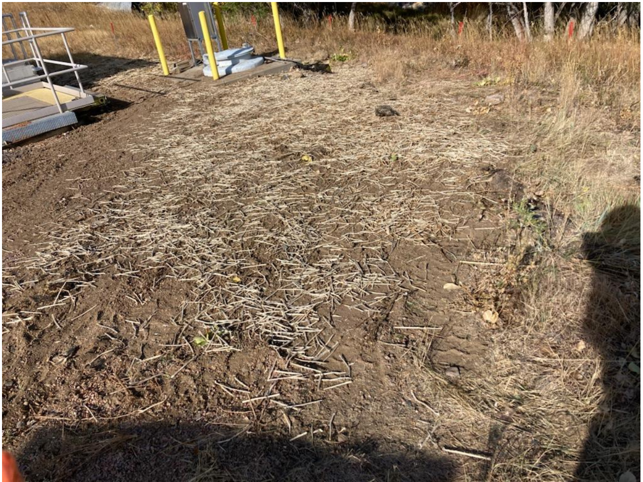
Photo 2. Work Area After Line Replacement and Backfill
