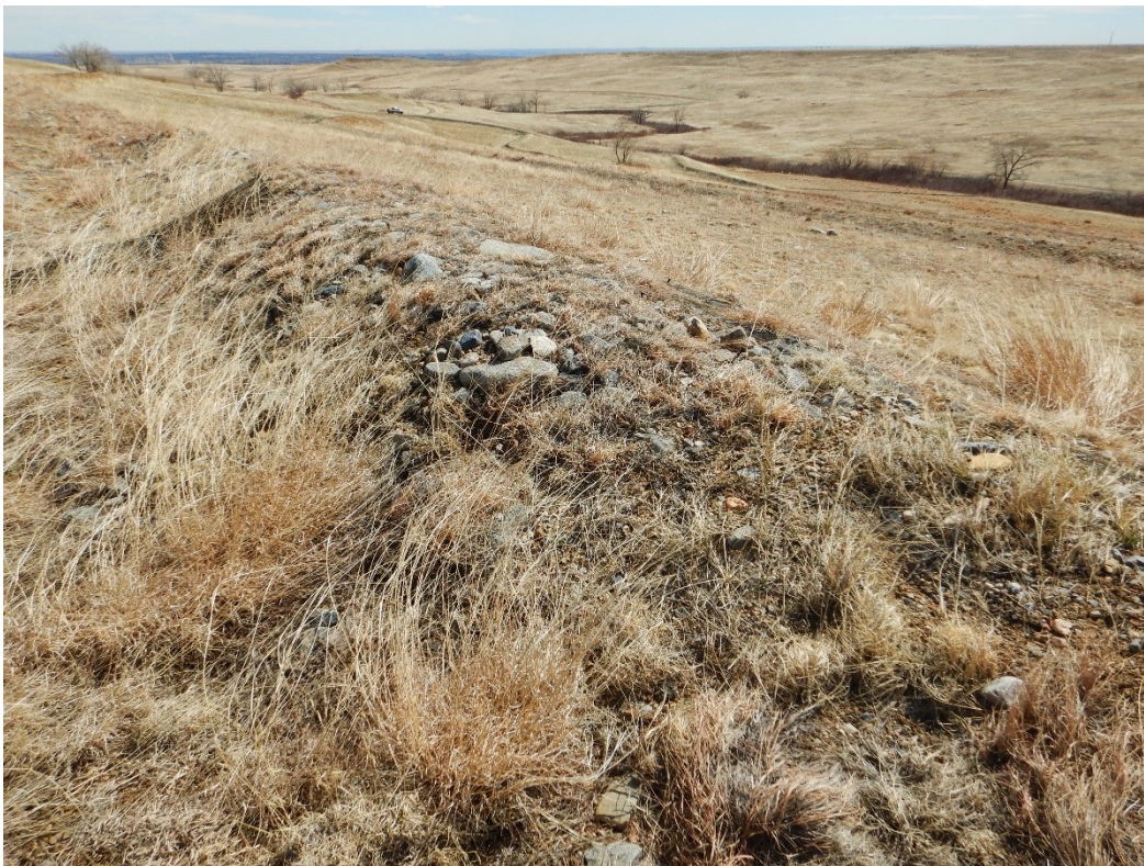
Figure 3. Looking Southeast at Berms 4–7 that Were in Good Condition
