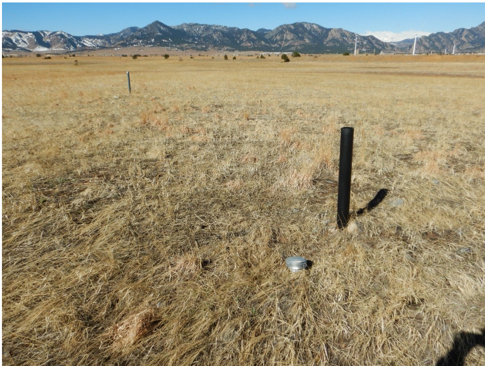
Figure 2. Looking West-Northwest at One of Four Caps that Have Fallen Off of their Gas Vents
