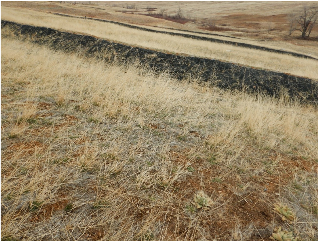
Figure 2. Looking South-Southeast at Berms 1–3 that Were in Good Condition
