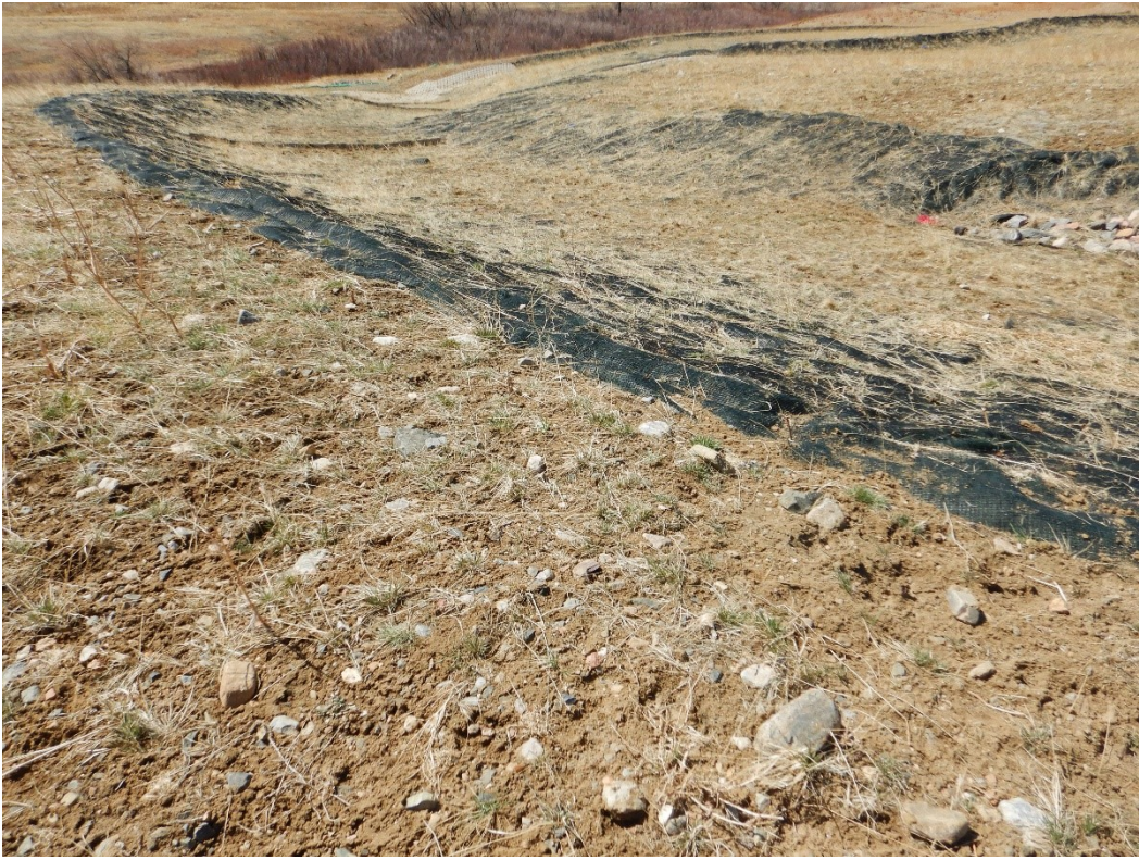
Figure 4. Looking South-Southwest at the EPC that Was in Good Condition
