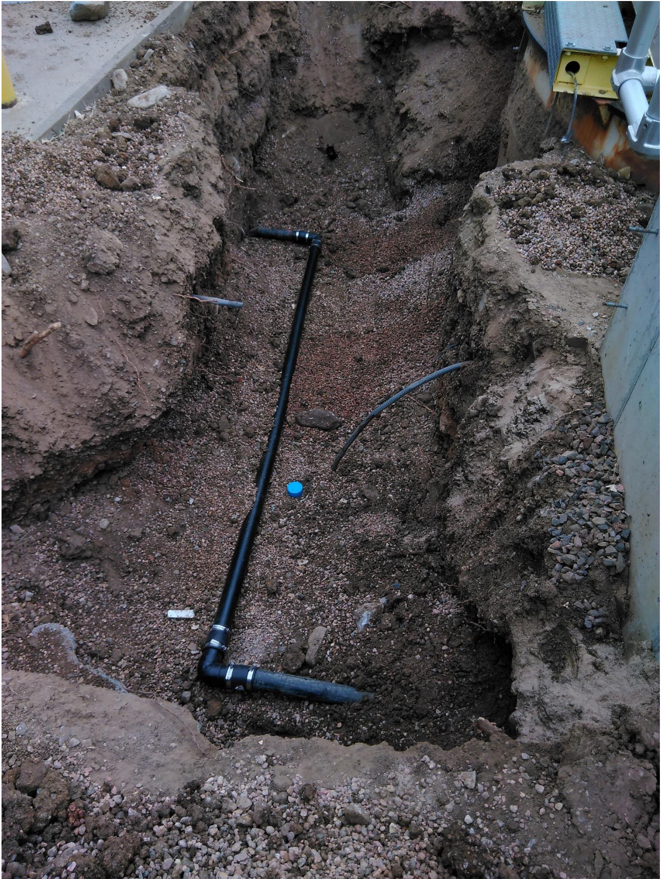
Photo 1. Excavation with New Effluent Discharge Line Installed
