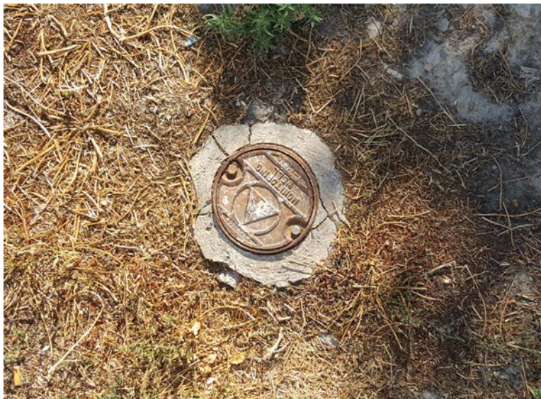
All observed wells appeared in good condition and well-maintained.
