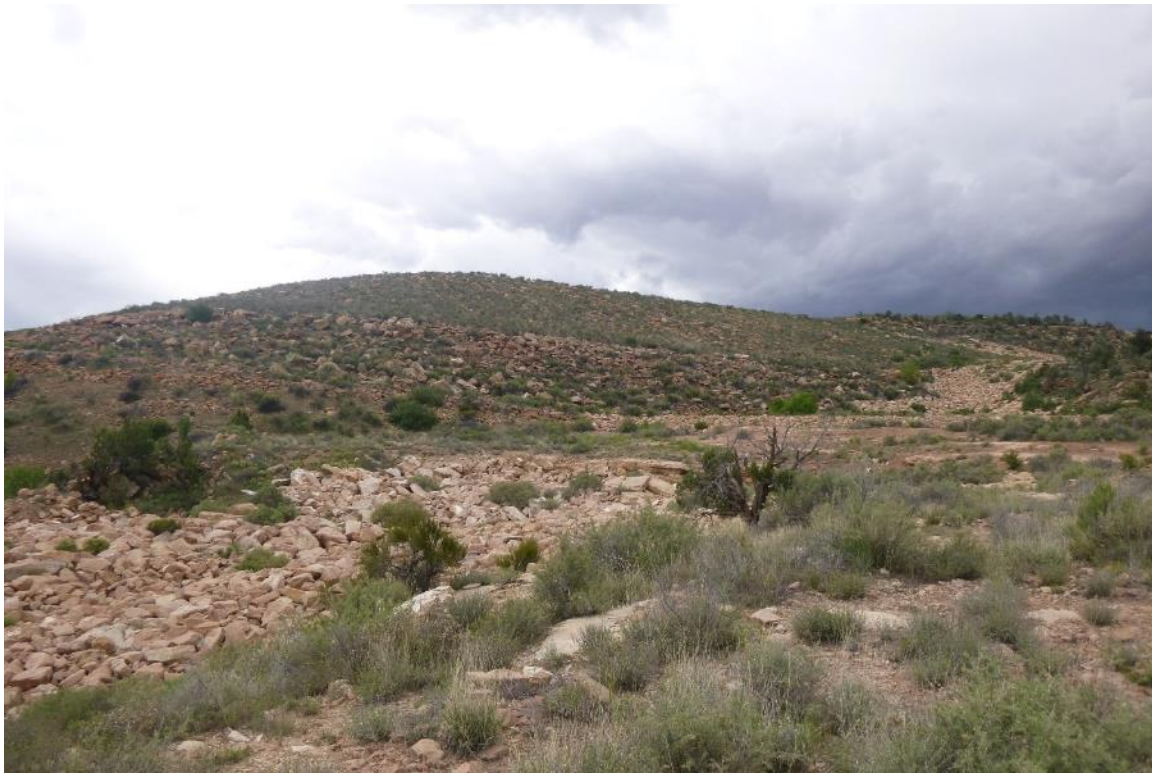
Drainage in foreground with Tailings Piles 1 and 2 in background.
