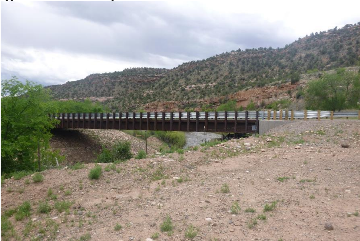
New County Road EE-22 bridge over the San Miguel River, looking toward F Block.
