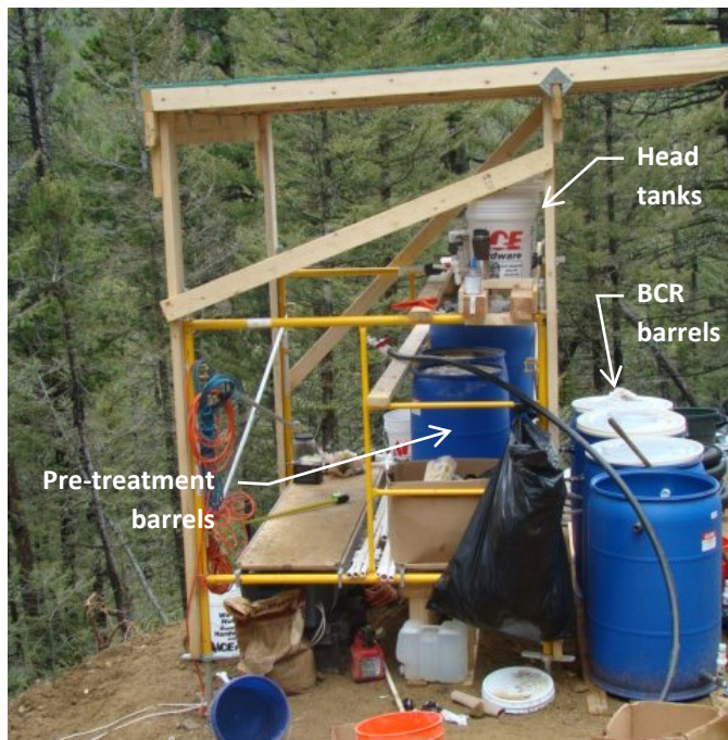
Exhibit 2-12. Completed scaffolding and platforms during treatment system construction.
