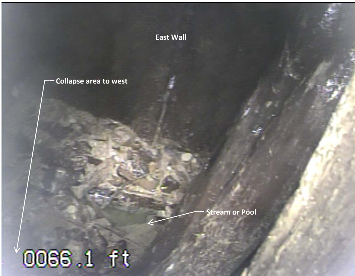
Exhibit 4-1. Bottom view of Tiger Shaft showing small stream or pool adjacent to collapse
