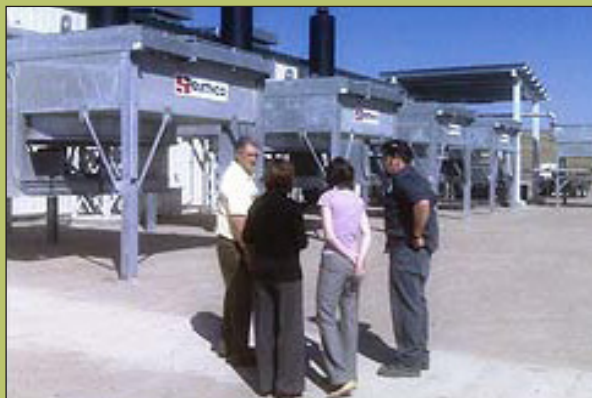
PICTURED: Tour of the Site's landfill gas-to-energy plant during its opening in 2008. (Source: City and County of Denver)
