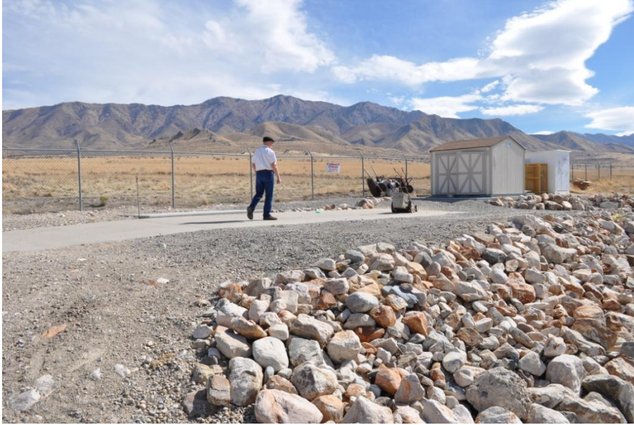
View towards SE corner of compound along eastern enclosure fence.
