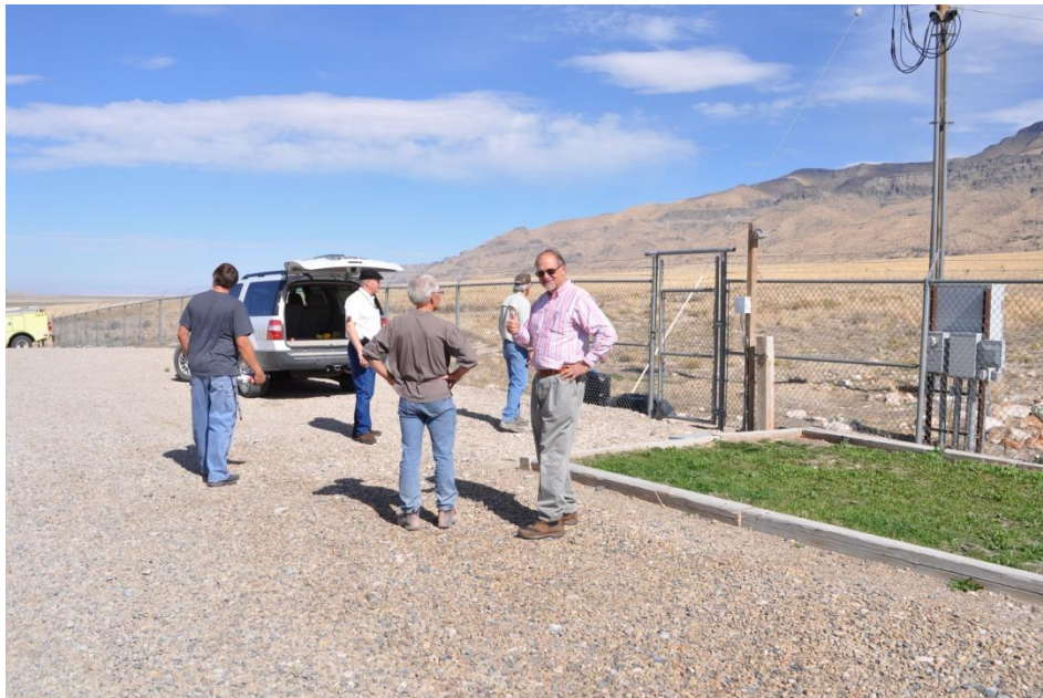
View along of pad area along eastern enclosure fence & gate near electrical panel.
