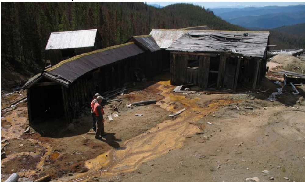
PHOTOGRAPH 3-3. Crystal Mine Structures
