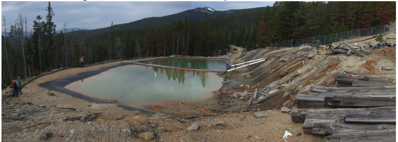
PHOTOGRAPH 1-2. Settling Ponds Constructed in the Mammoth Dump
