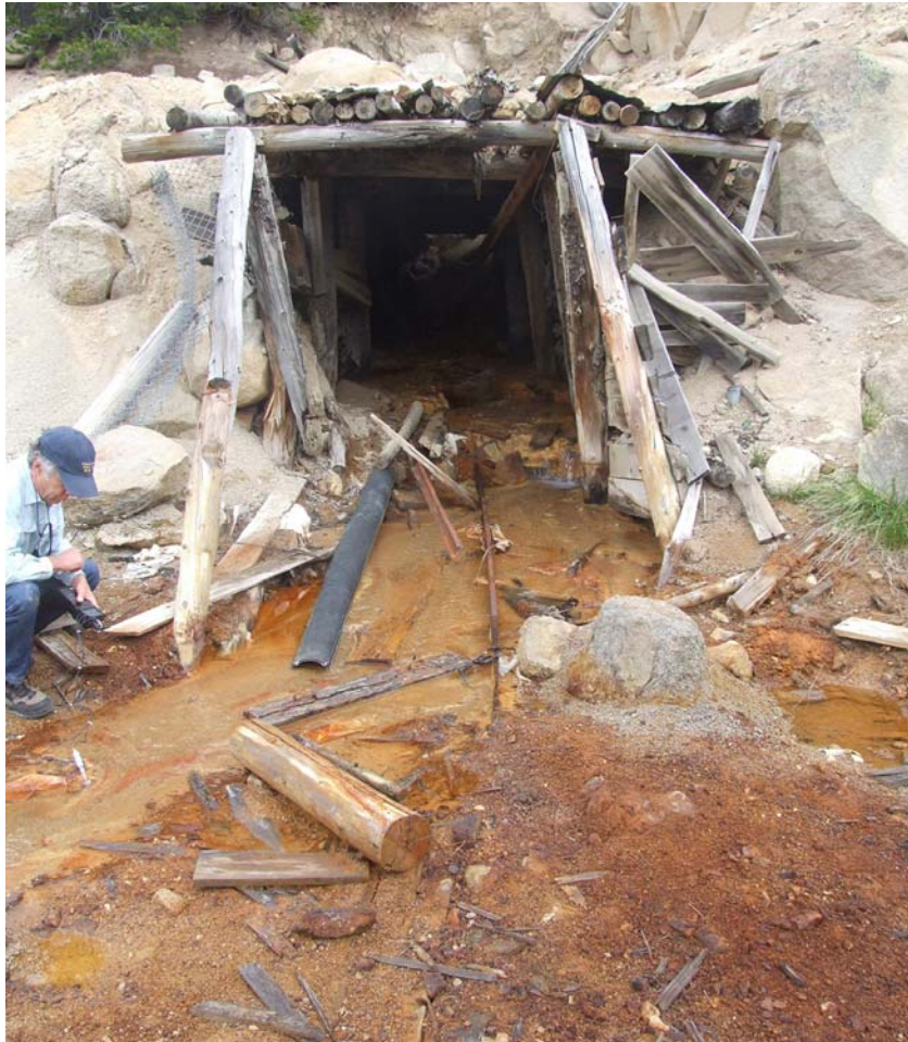
PHOTOGRAPH 1-3. Iron Oxide Staining Representative of AMD
