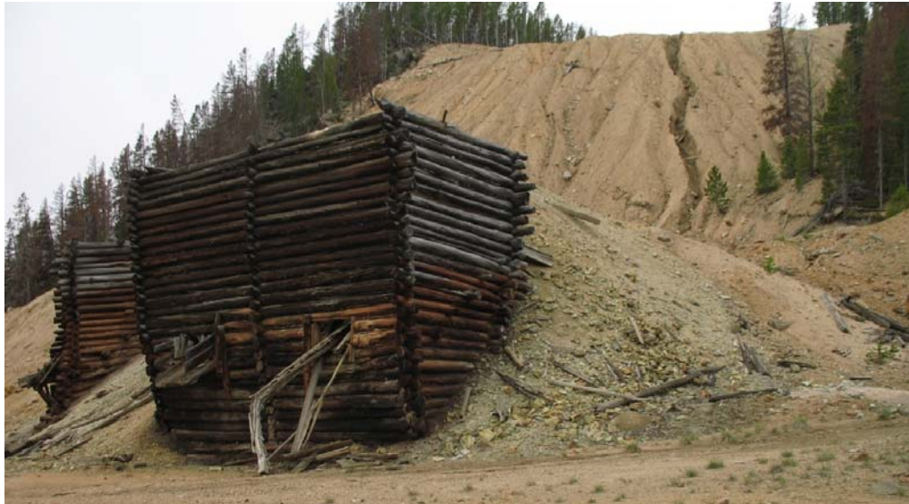
PHOTOGRAPH 3-4. The Crystal Dump at the East End of the Trench (Background) Covering the Upper Crystal Mine Portal and the Twin Ore Bins Dump (Foreground)
