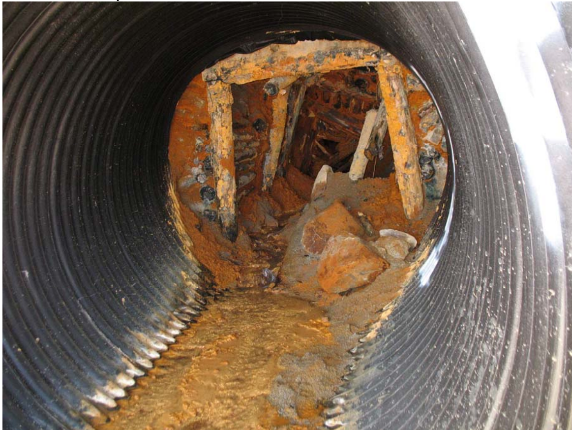
PHOTOGRAPH 3-5. Crystal Mine Lower Portal Current Condition
