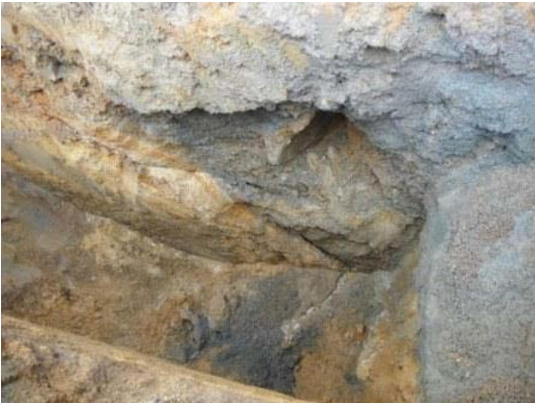
Photo 2: Seepage from two fractures in weathered granitic rock, approximately 6 feet bgs.
