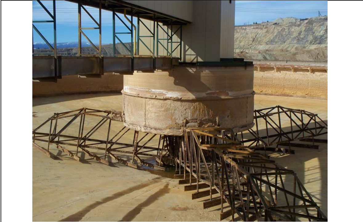
Photo 5. Clarifier with rakes visible (drained for maintenance).
