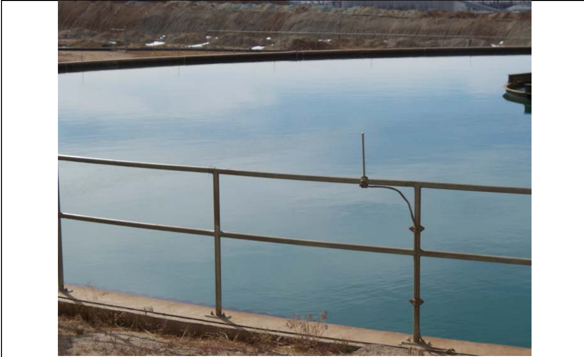
Photo 9. Looking across clarifier.
