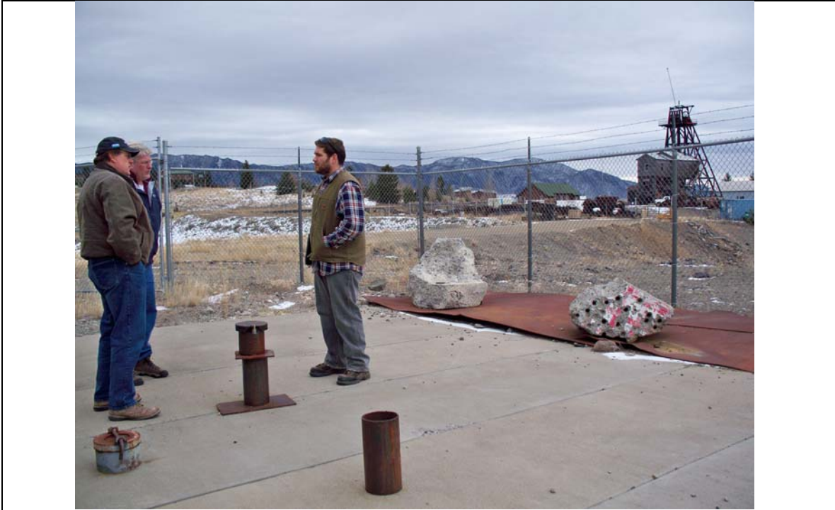
Photo 10. Orphan Boy mine shaft cover and monitoring well.
