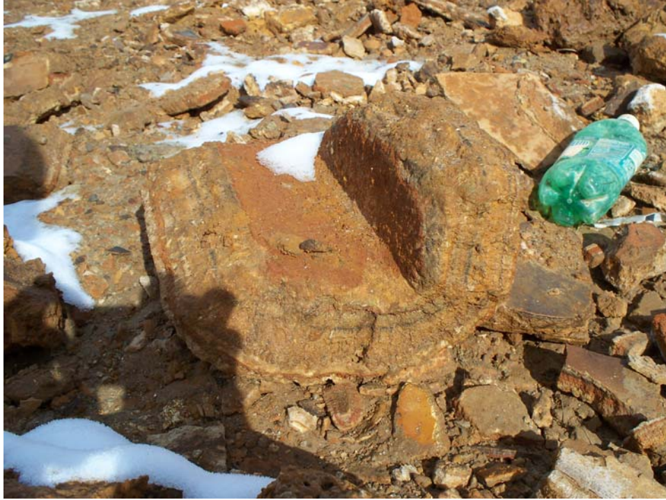
Photo 7. Large block of scale removed from vessel wall, note thickness.
