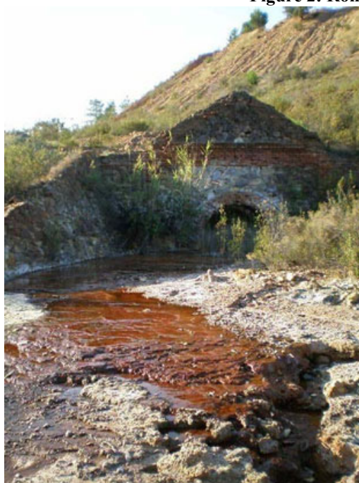
Figure 2: Roman Portal with Acid Rock Drainage – Spain
