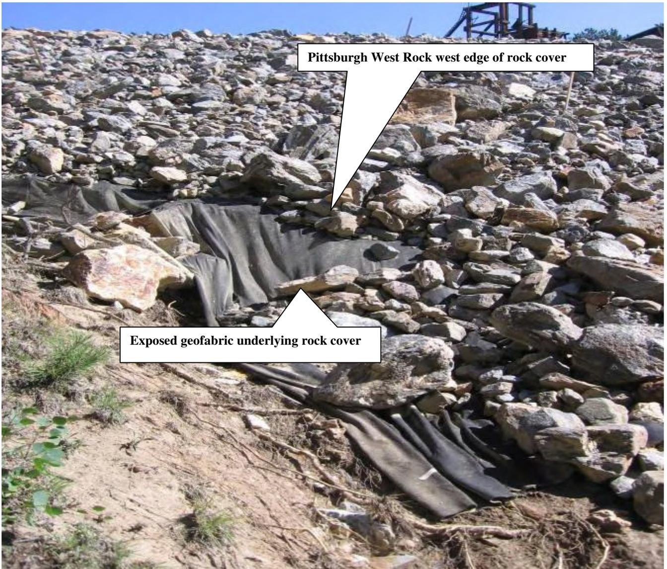
**View to east along the Pittsburgh Waste Rock Pile where scouring exposed geofabric underlying the rock cover.**
