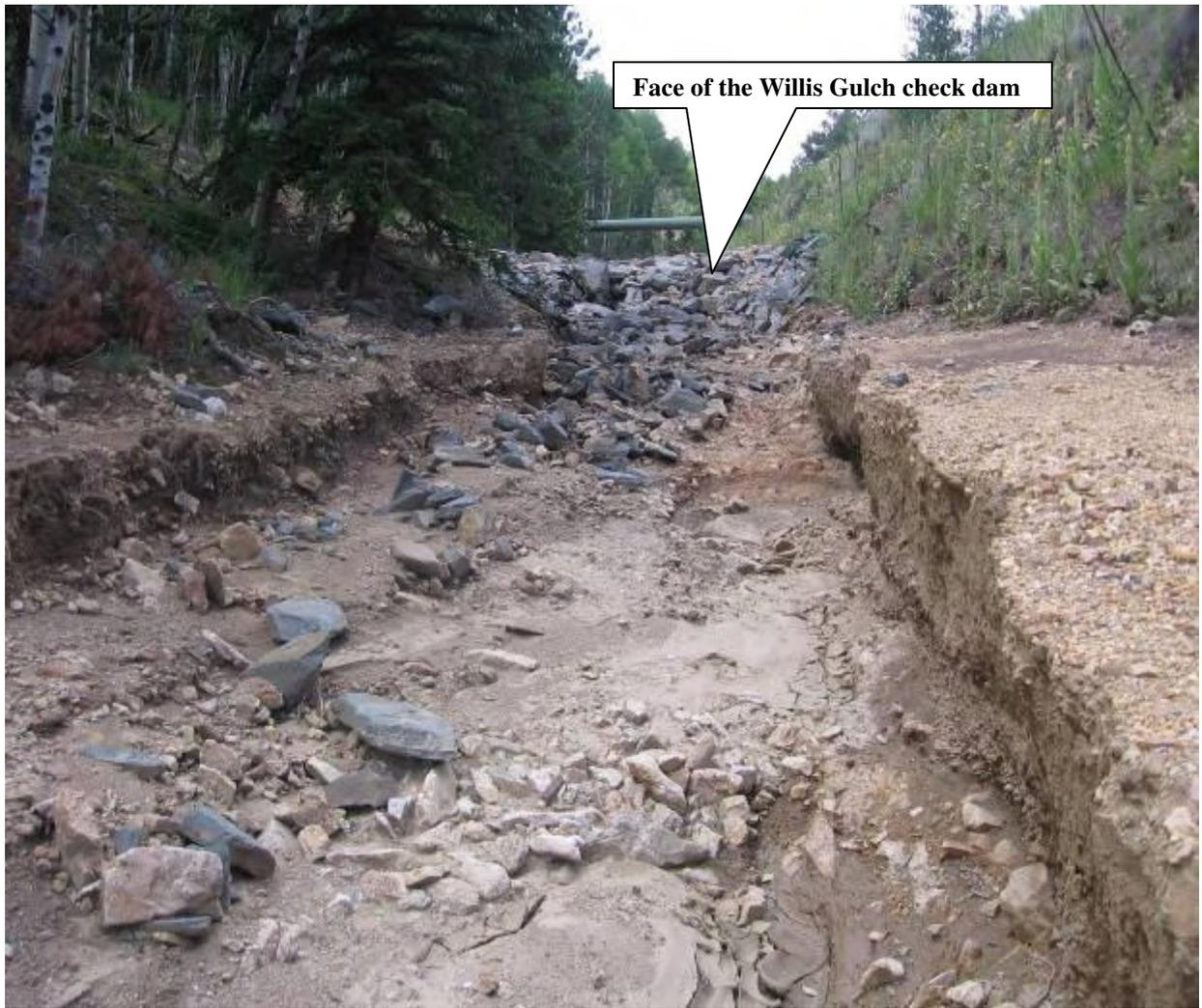
**View to west at the Willis Gulch check dam constructed during the Phase I OU 4 activities. The July 25-26, 2009 storm event resulted in the failure of the face of the dam. Dark gray rocks in the lower left hand corner of the picture were transported from the face of the dam during the storm event. The channel scour is approximately two feet deep, whereas the channel was level across the channel width after construction of the dam.**
