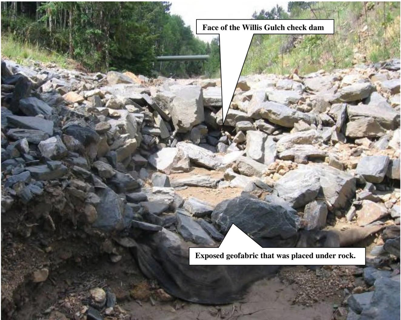
**View to west at the Willis Gulch check dam. The July 25-26, 2009 storm event resulted in the failure of the face of the dam and the filling of the upstream face of the dam with sediment. The center of the picture shows the scouring to the face of the dam during the storm event flow in Willis Gulch. At this point any water will flow directly over the dam without slowing down and sediment will not be retained behind the dam.**
