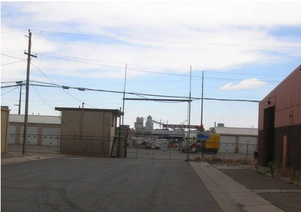
OU2 – Jerome Maintenance Yard CDOT – 2300 West 11 th Avenue
