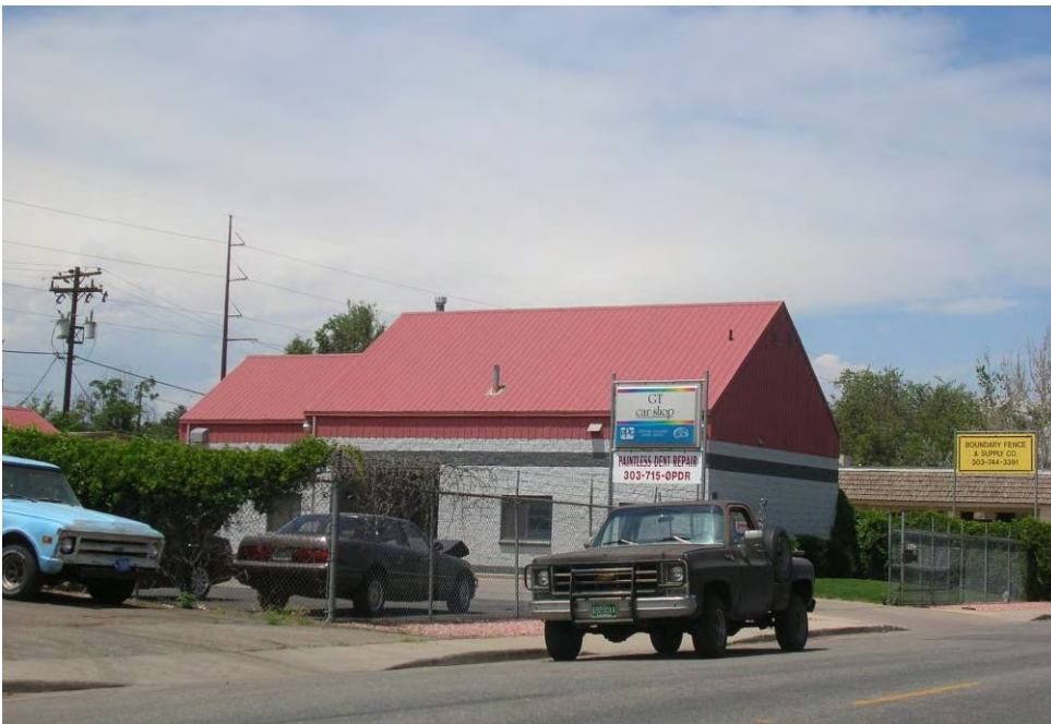
OU3 – GT Car Shop – 1235 South Jason Street
