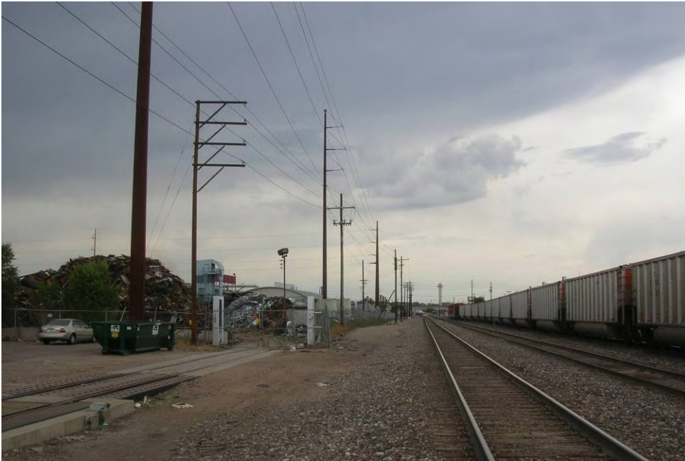
OU2 – Burlington Northern Railroad ROW – Between 10 th and 11 th Avenues
