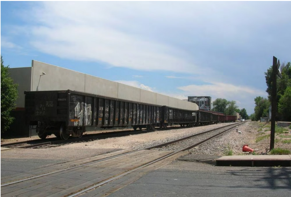
OU3 – Central and Sierra Rail Road ROW – Between West Louisiana and West Florida Streets.
