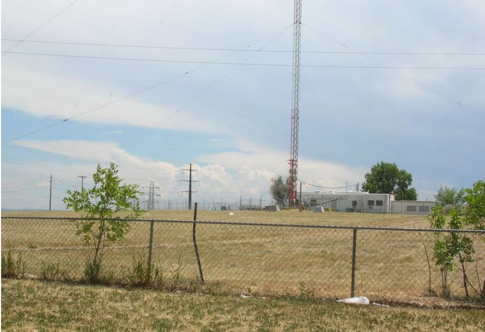
OU6 – Public Service Company – South Pecos Street and West Arizona Avenue
