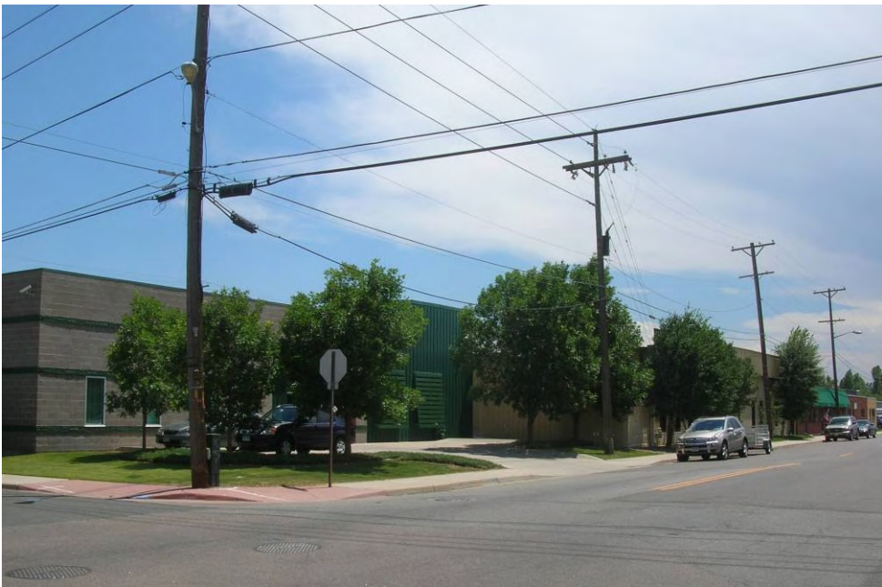
OU3 – Various Offices – 1300 South Jason Street
