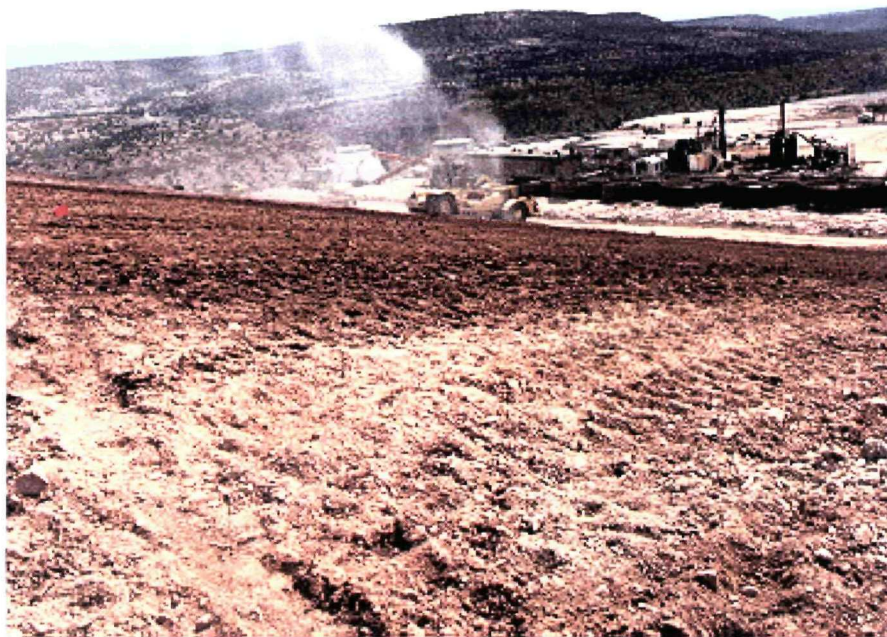
Photo 4.4-2: Regrading of Tailing Pile #1-2 Slope, B-Plant in Background, May 1989
