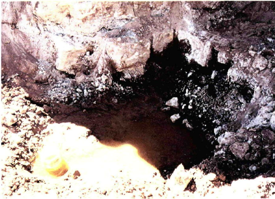
Photo 4.4-10: Tailings Pile #1-2, Ground Water Seepage, October 1999
