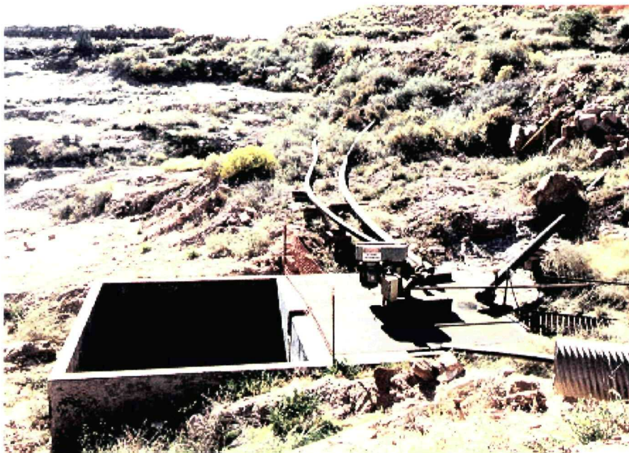
Photo 5.1.2.5-1: Toe Drain Collection Sump#2 and Associated Piping, October 1999
