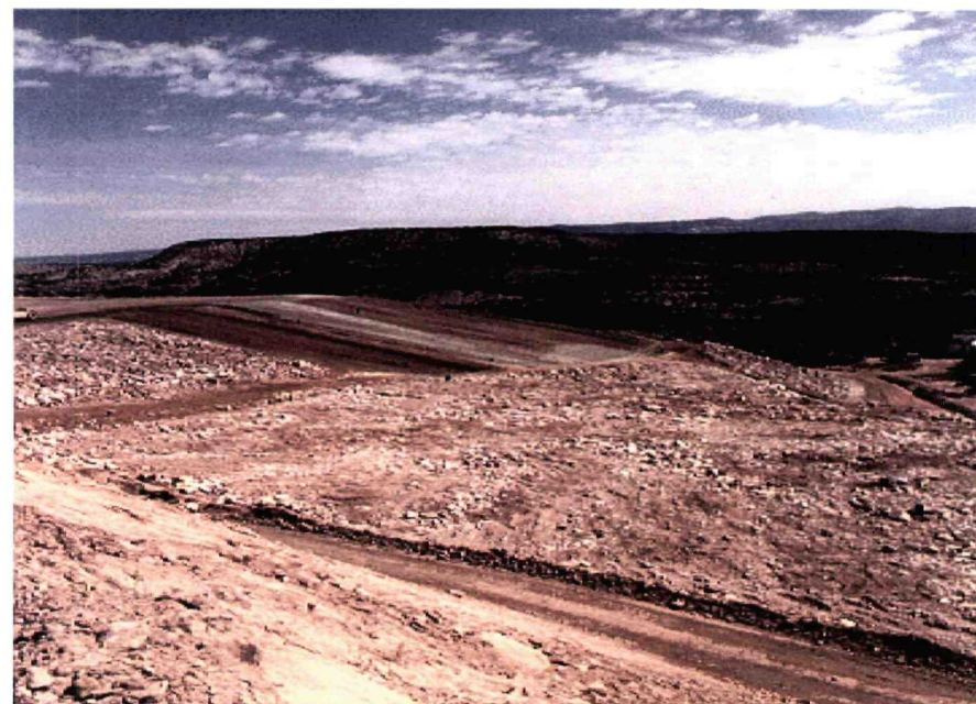
Photo 4.4-1: Regrading and Contouring of Tailing Pile #1-2 Slope, May 1989
