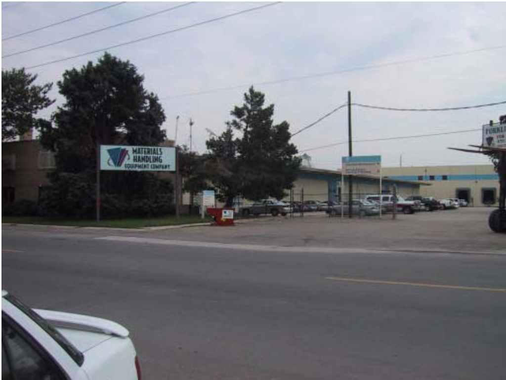
1740 West 13 th Avenue – Materials Handling Inc.
