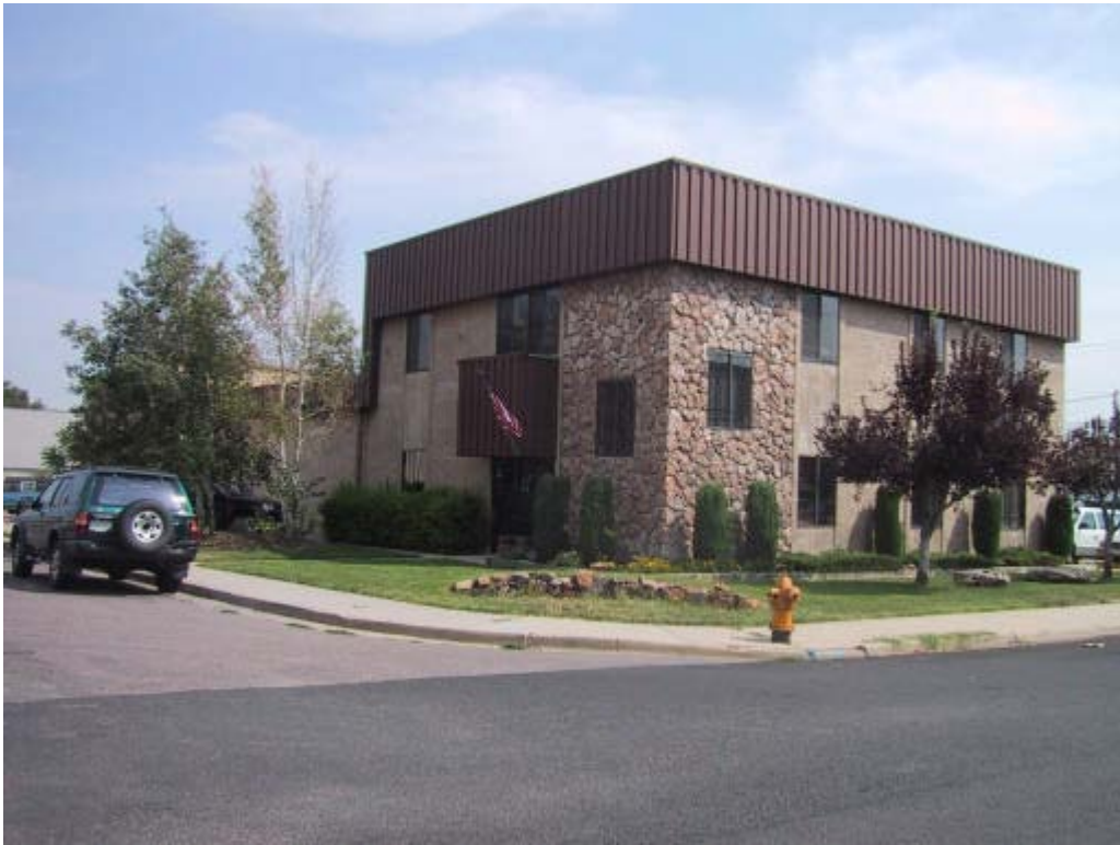
1298 South Kalamath Street - Creative Illumination Inc.
