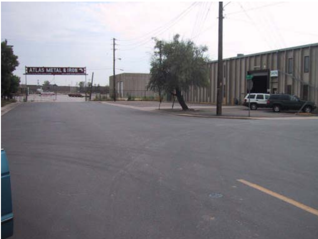
1900 West 12 th Avenue (Flame Spray, Inc.) on right and 1100 Umatilla Street (formerly DuWald Steel) on left.
