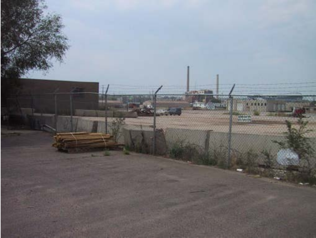
1001 South Tejon Street - Air Conditioning, Inc. with 1100 Umatilla in background. OU2 (continued)
