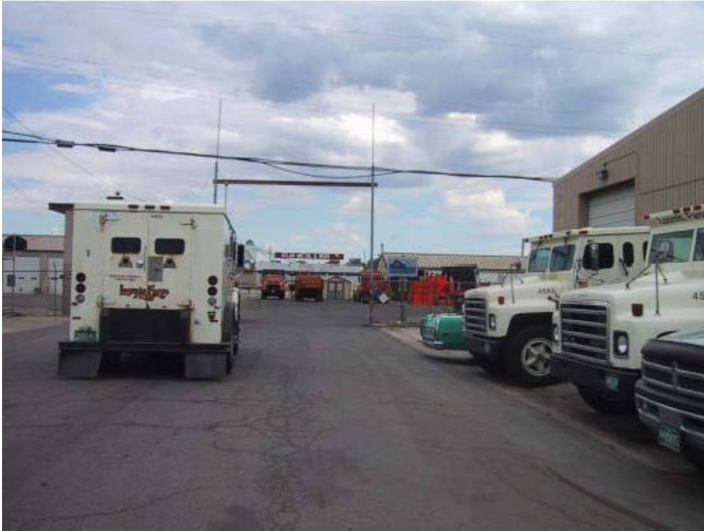
2300 West 11 th Avenue - Colorado Department of Transportation Jerome Maintenance Yard with 1100 Umatilla in background.
