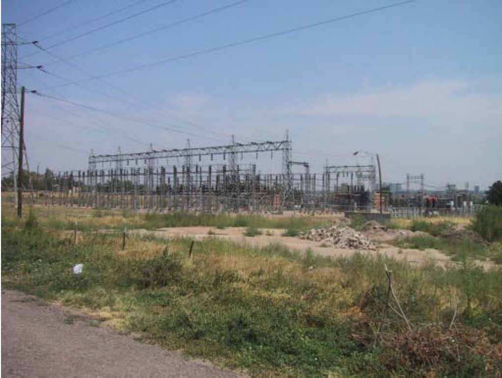
South Pecos Street and West Arizona Avenue - Public Service Company
