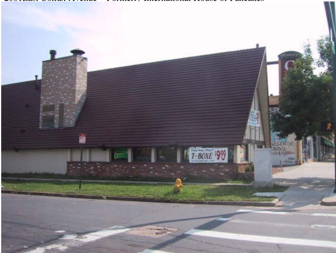
2001 East Colfax Avenue – Formerly International House of Pancakes
