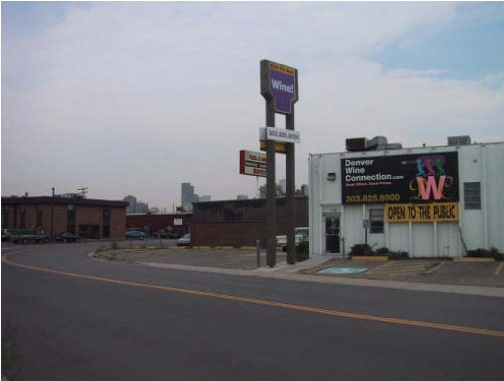
1190 Yuma Street - Denver Water Department
