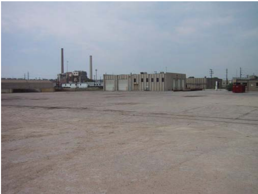
1100 Umatilla Street - formerly DuWald Steel now Atlas Metals
