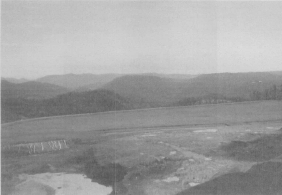
Photo No. 1 Top of Ruby Repository, Seen from Heap Leach Pad View to East
