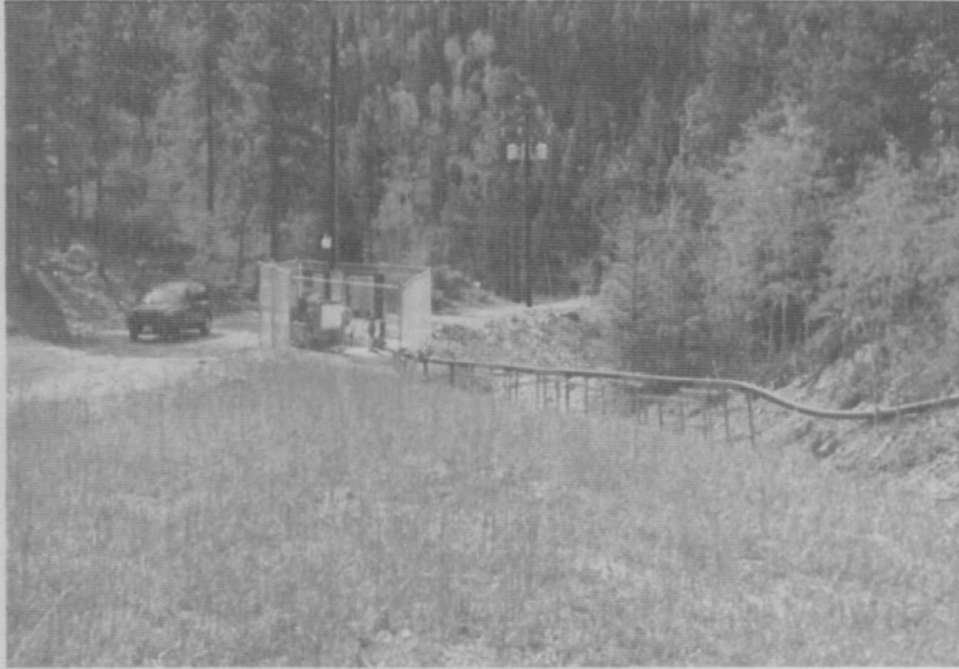
Photo No. 5 Hoodoo Gulch Lift Station View to South
