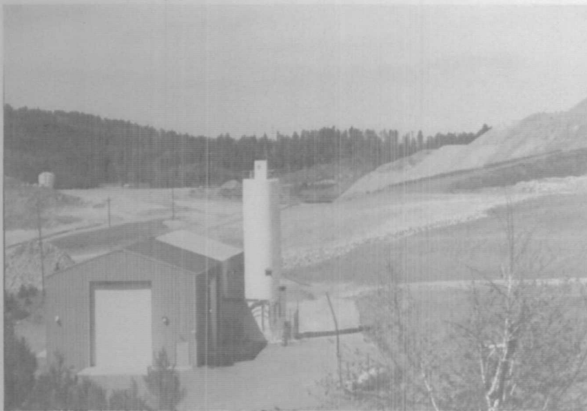
Photo No. 4 Water Treatment Plant View to West
