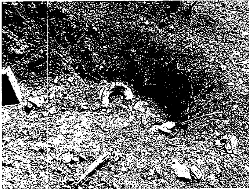
Figure 7 – Blocked culvert at the Tramway drainage in Belden.
