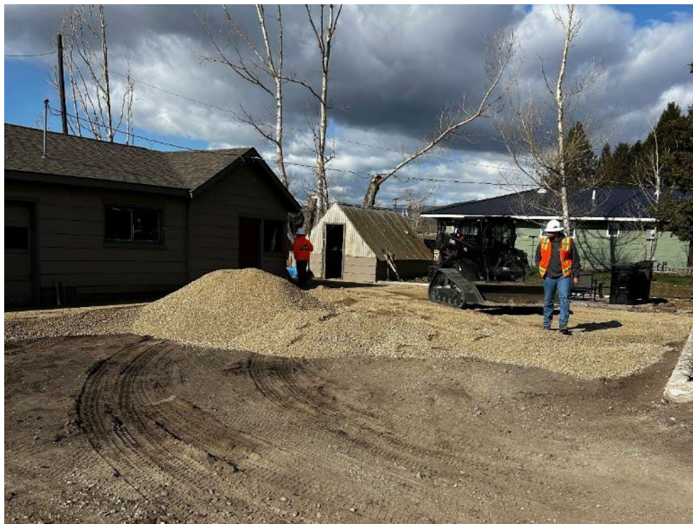
Work being done for residential yard cleanup (OU16)
