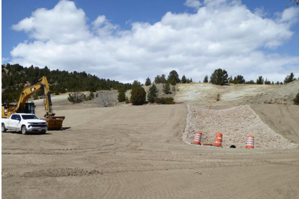
McCurdy sediment pond under construction (OU4, RDU-2)
