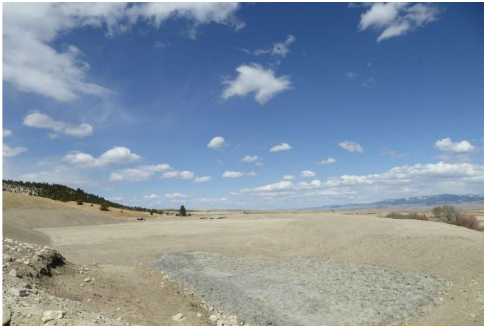
Lost Creek North Sediment Pond under construction (OU4, RDU-2)
