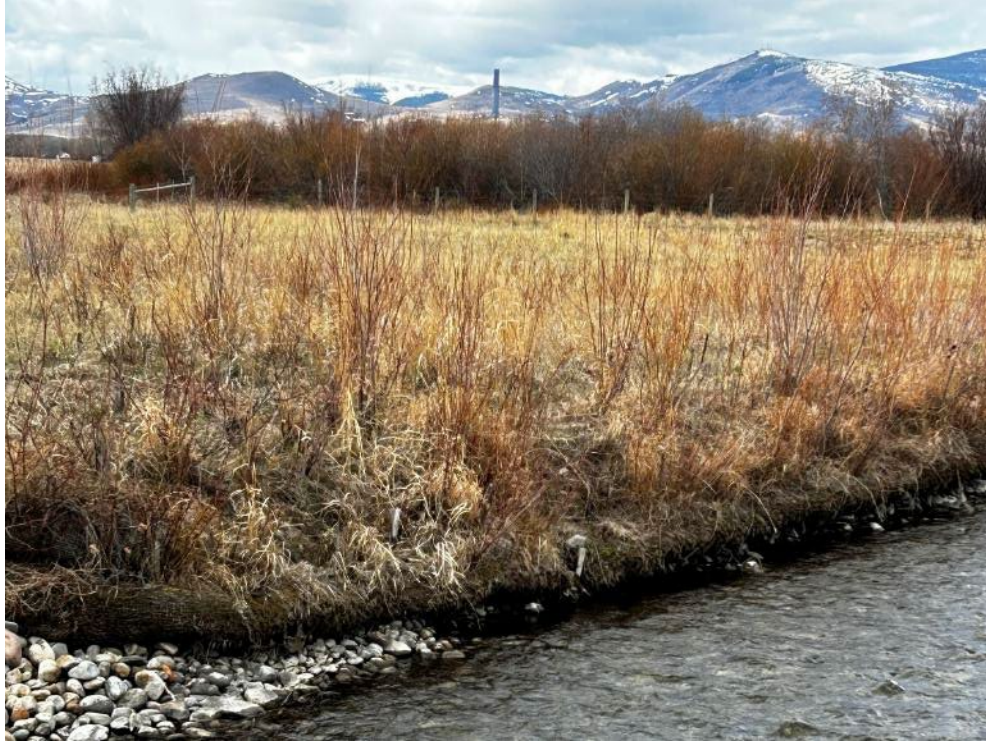
Bank stabilization at Warm Springs Creek (OU4, RDU-10)
