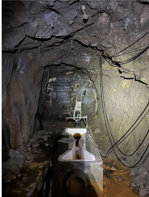
Level 1 bulkhead and flume
