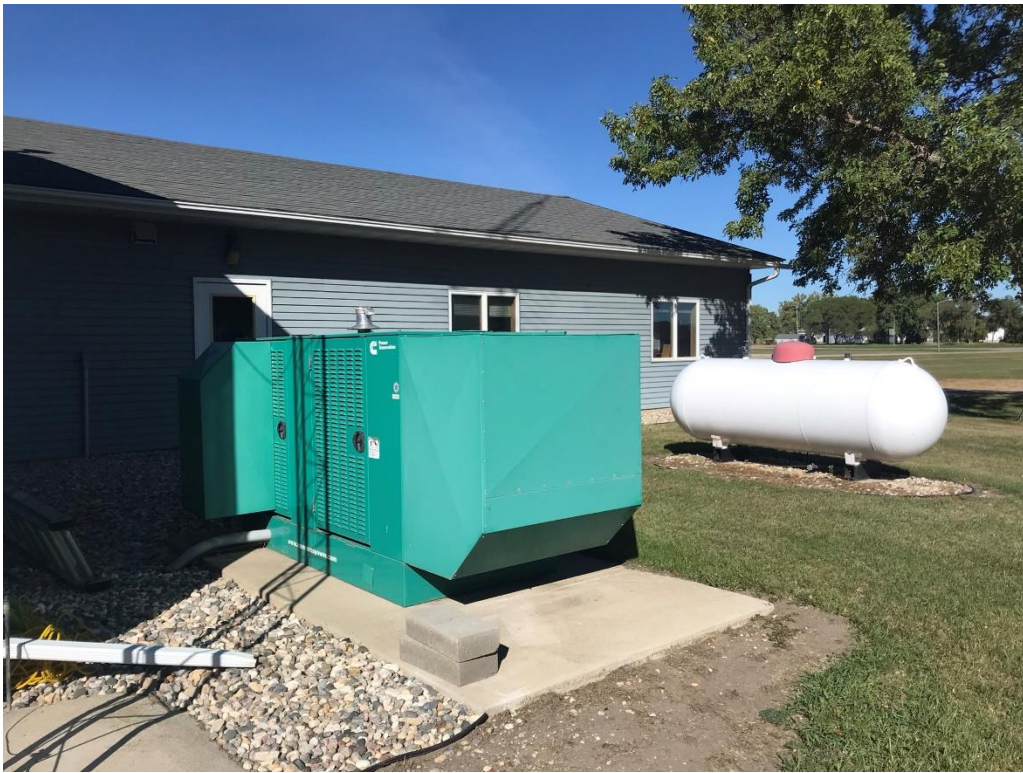
Emergency generator for geothermal unit, located outside SEWUD building
