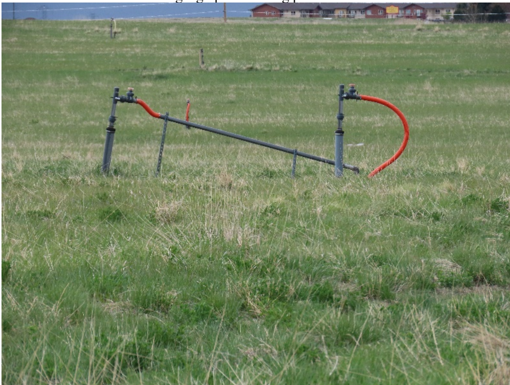
Landfill gas extraction system, typical well
